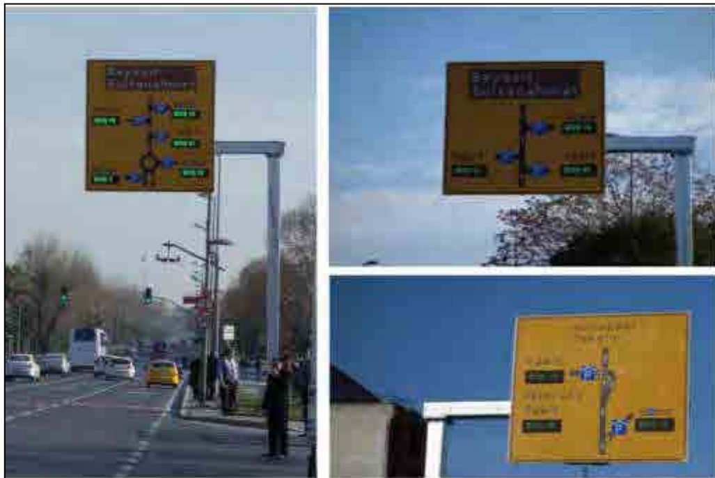
Figure 2.1.6 Parking Information Service through Information Boards
