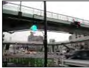
Overpass and Signalization
