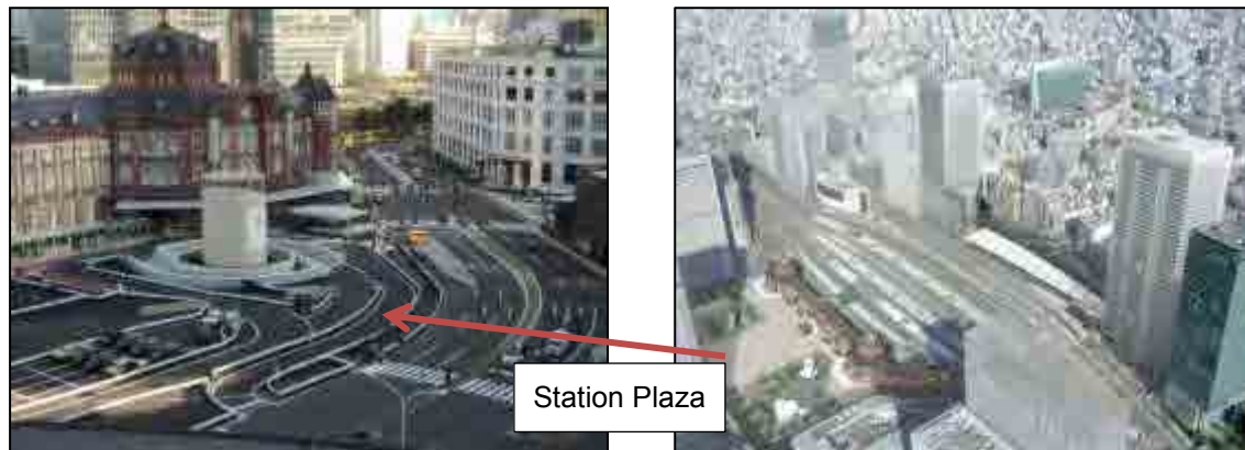
Photo 1.3.1 Yaesu-side Station Square and Bird's Eye View of Tokyo Station Area
