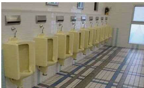
▲ Maintain clean toilet
