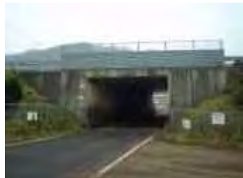
Figure 5.5-6 Example of Box Culvert
