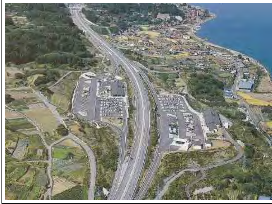
Figure 4.4-1 Image of Rest Area
