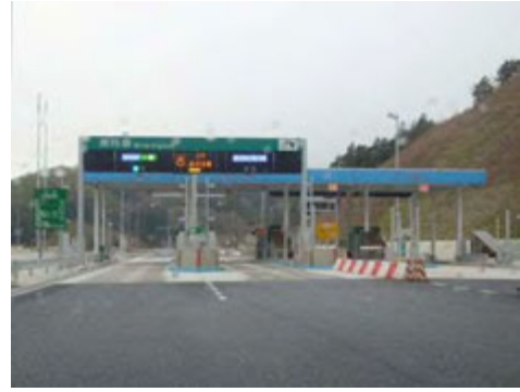
Figure 7.2-2 ETC Toll Gate
