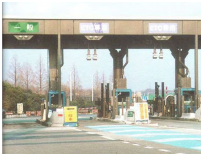
Figure 10.1-1 ETC Toll Gate
