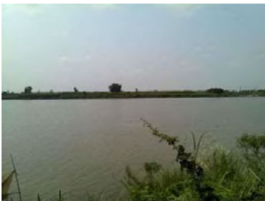
Figure 4.2-12 Crossing Point of RR3 over Mekong River: Photo from East Side
