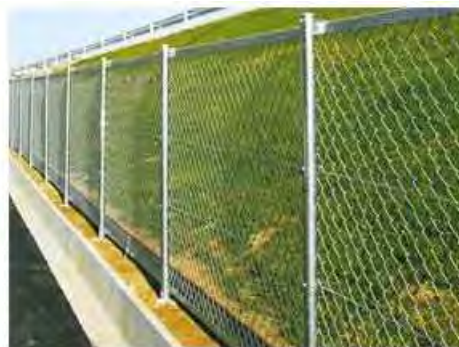
Figure 5.6-13 Example of Fence
