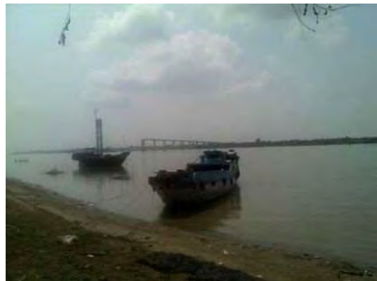
Figure 4.2-11 Crossing Point of Route B over Mekong River: Photo from East Side
