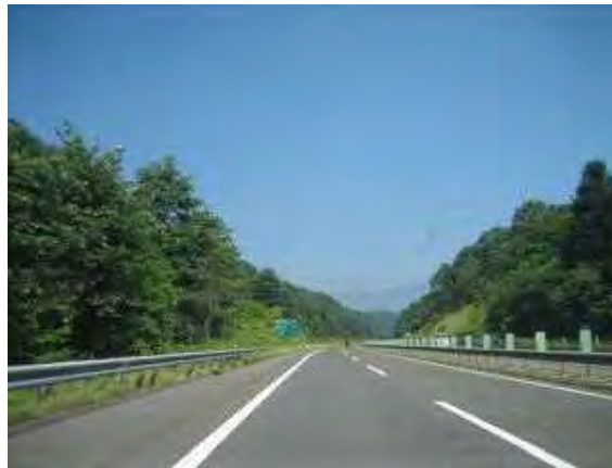
Figure 5.6-11 Photo of Guardrail
