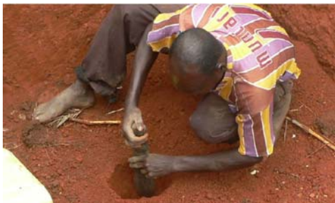
Drilling of test hole
