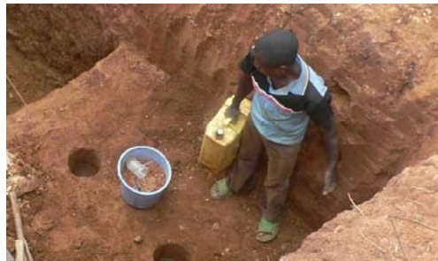
Water splinkling and feeding to test hole
