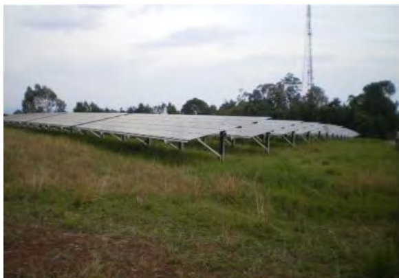
4,000 of solar panels with inclination angle of 10°±, made in USA
