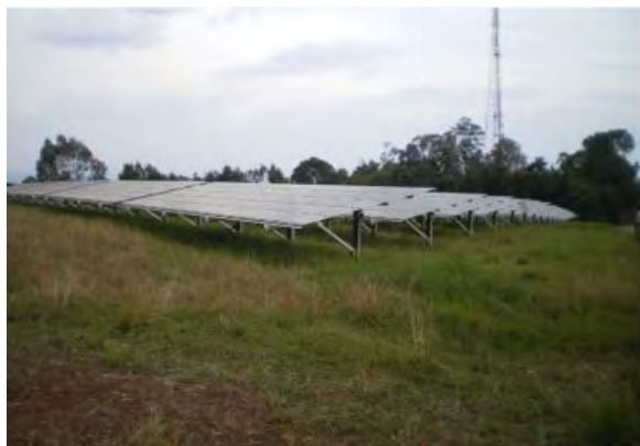
4,000 of solar panels with inclination angle of 10^{\circ} \pm , made in USA
