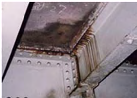
No 3: Member Girder
