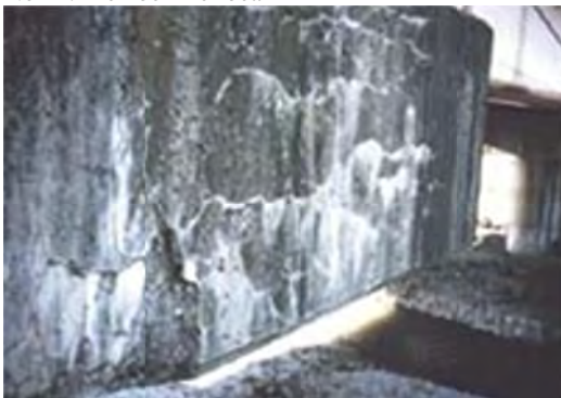
No 11: Member Pier beam
