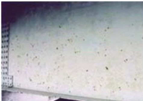
No 5: Member Girder
