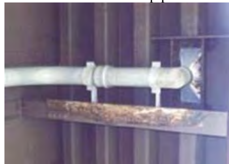
P 5: Member Drain pipe
