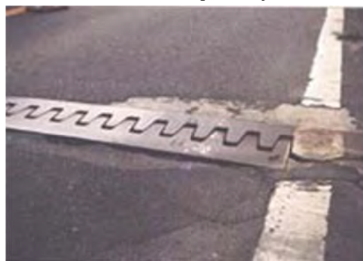
P 2: Member Expansion joint
