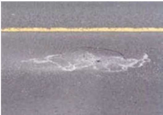
P 3: Member Pavement
