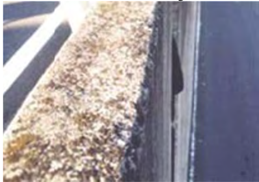
P4: Member Railing
