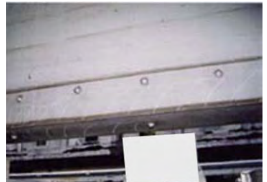
No 2: Member Girder
