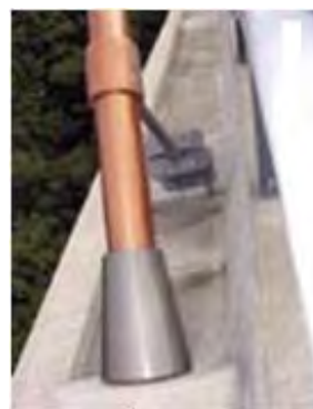
P18.4 Anchor of cable Stay Bridge (good)
