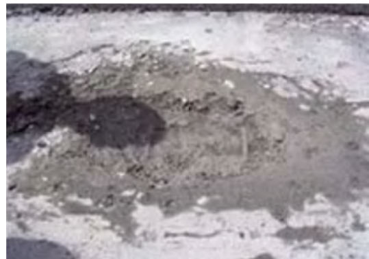
2) Floor deck upper part changed to sand
