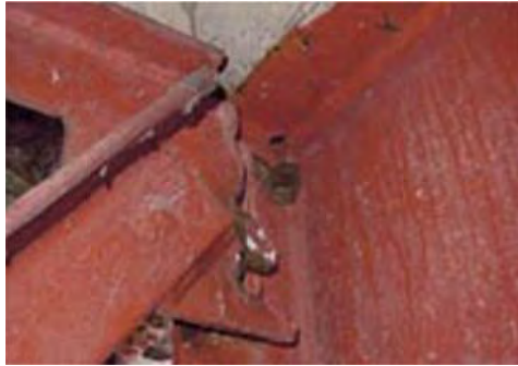
No 1: Member Diagonal bracing
