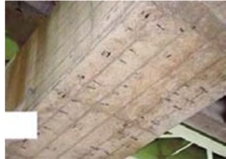
No 4: Member Pier beam
