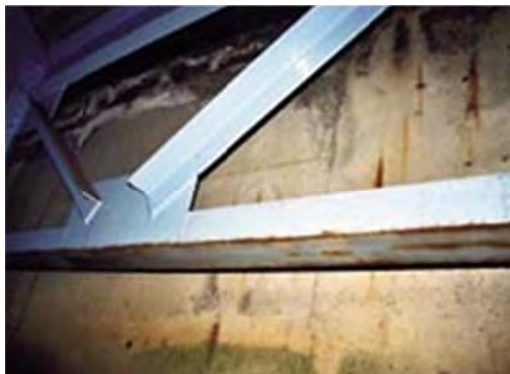
No 5: Member Cross beam
