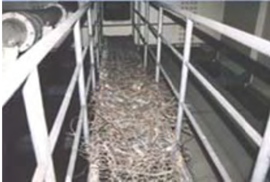
P7: Member Foot bridge
