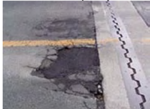
P 4: Member Expansion joint
