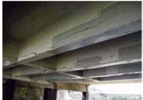
No 6: Member Girder
