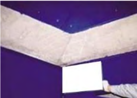
No 3: Member Floor deck
