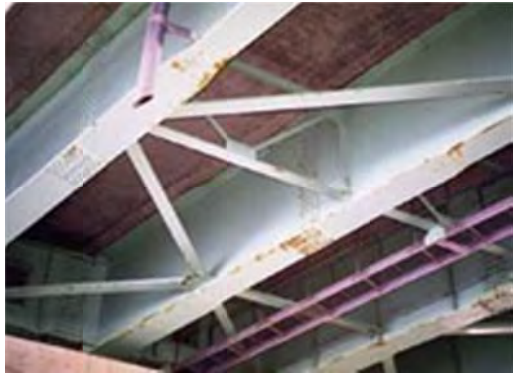
No 1: Member Main girder
