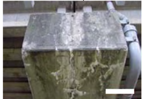
No 12: Member Beam at pier
