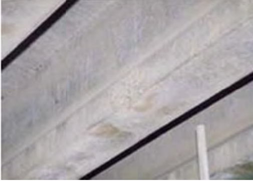
Remark: Pylon wall
