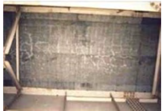
No 2: Member Floor deck
