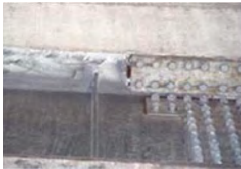
No 9: Member Girder
