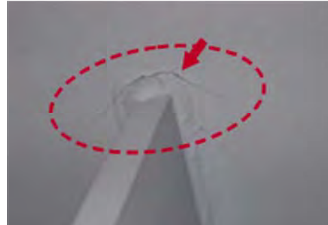
No 2: Member Steel deck plate
