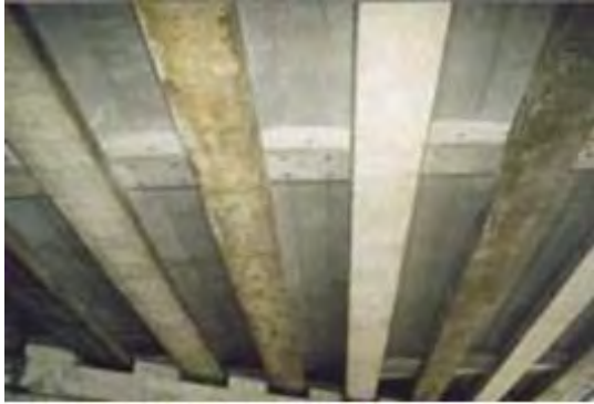
P 1: Member Girder
