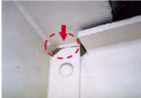
No 1: Member Girder
