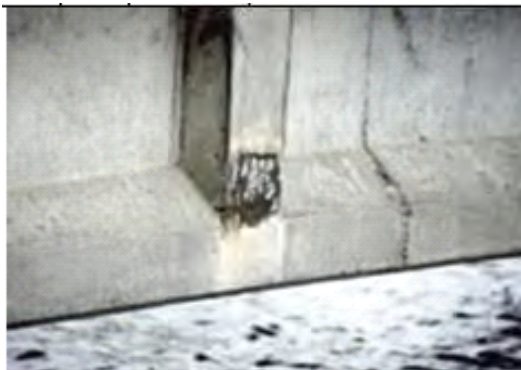
P 3: Member Girder
