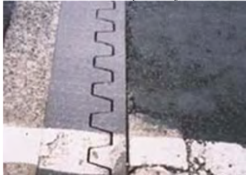
P 3 Member Expansion joint
