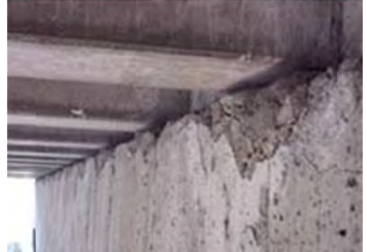
Remark: Pylon wall
