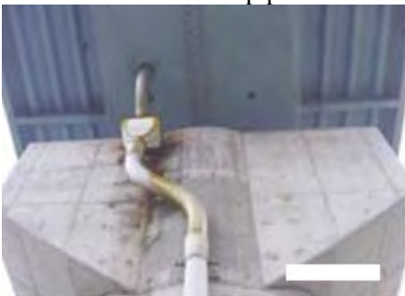
P 4: Member Drain pipe
