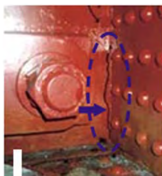
No 5: Member Girder connecting
