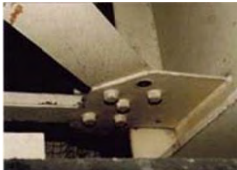
No 3: Member Lower bracing
