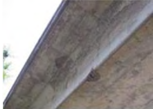
P 4: Member Floor deck
