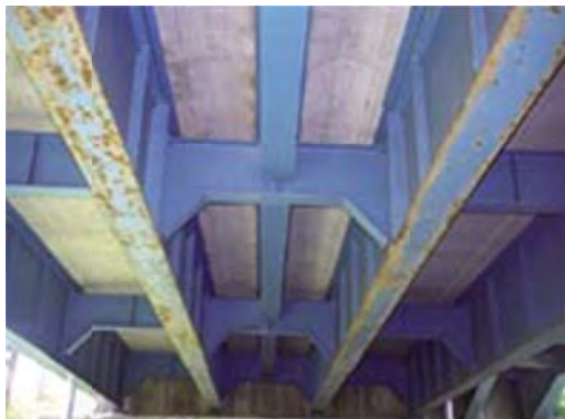
No 3: Member Girder
