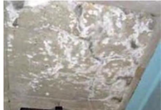
No 6: Member Floor deck
