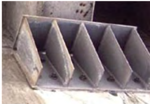
No 11: Member Bridge prevent collapse system
