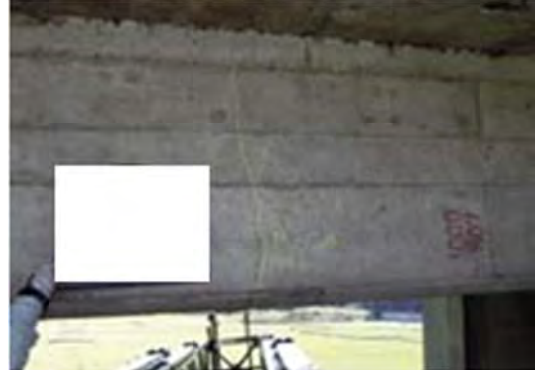
No 8: Member Girder
