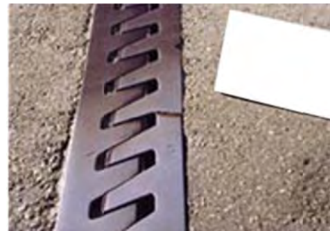
No 4: Member Expansion joint
