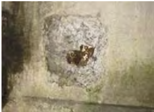
P 3: Member Girder
