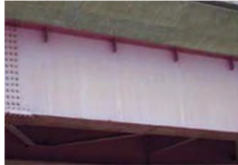
No 2: Member Girder
