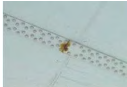
Outside of box girder
