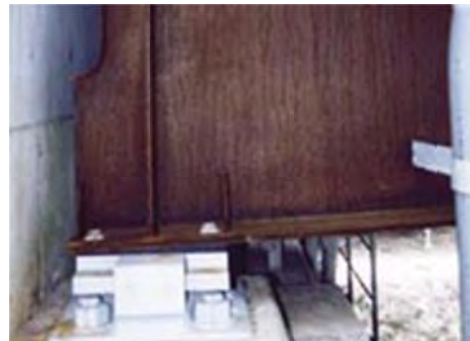
No 10: Member Girder
