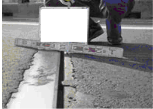
P 2 Member Expansion joint
