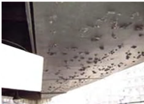
No 3: Member Girder
