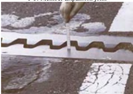
P 3: Member Expansion joint
