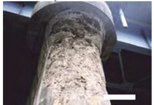
No 12: Member Pylon wall
