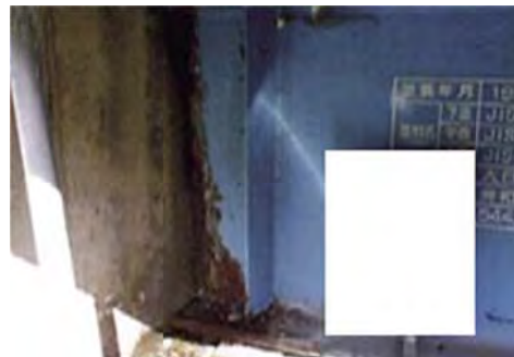
No 6: Member Girder
