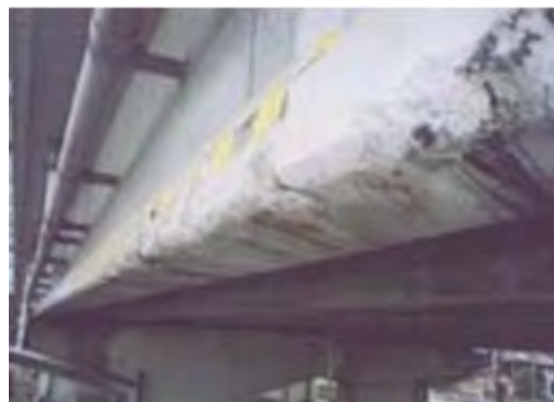
P 2: Member Girder
