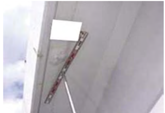
No 2: Member Floor deck
