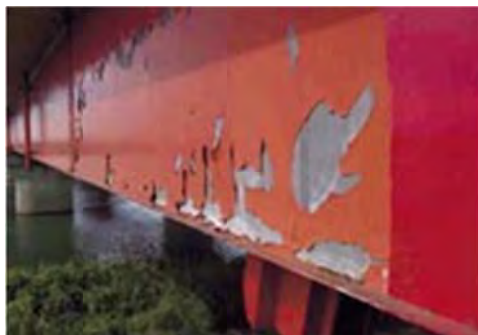
No 5: Member Girder
