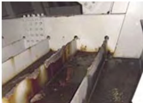
Inside of box girder
