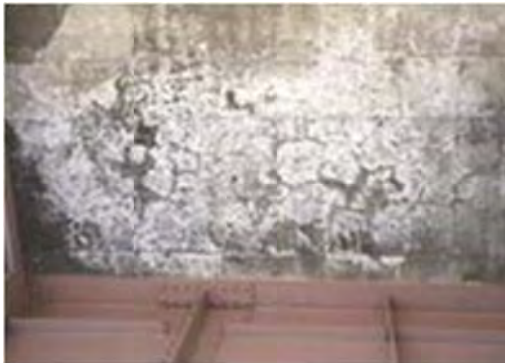
No 9: Member Floor deck
