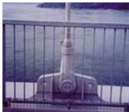
P18.6 Hanger anchoring portion in suspension bridge (good)
