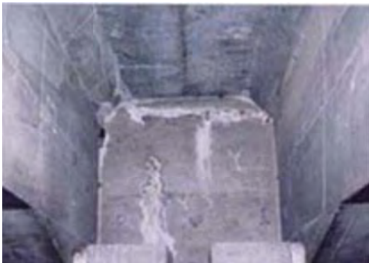
No 5: Member Cross beam
