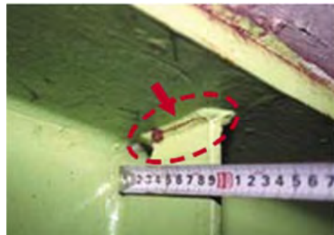
No 4: Member Girder
