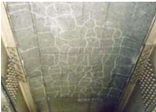
No 5: Member Floor deck
