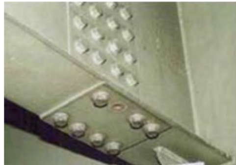
No 4: Member Cross beam
