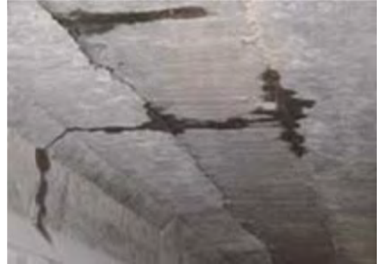
No 2: Member Floor deck
