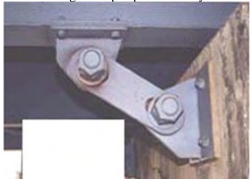
P 6 Bridge collapse prevention system
