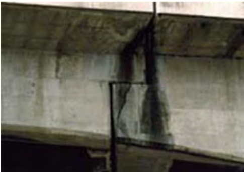
No 3: Member - Girder
