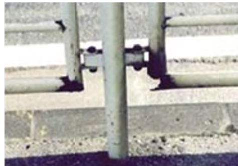
No 4: Member Railing
