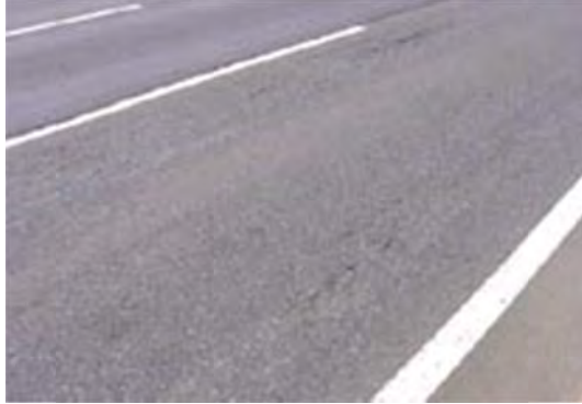
P 1: Member Pavement
