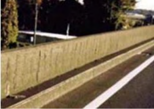
No 1: Member Handrail
