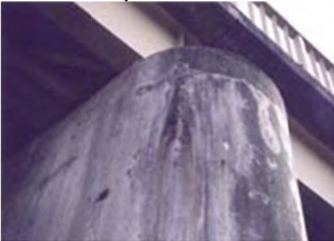
No 9: Member Pylon wall
