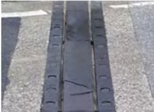
P 3: Member Expansion joint
