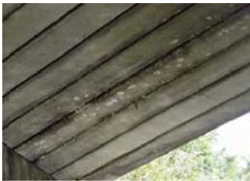
P8.3 Between floor deck beam
