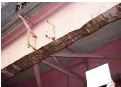
P 1: Member Girder
