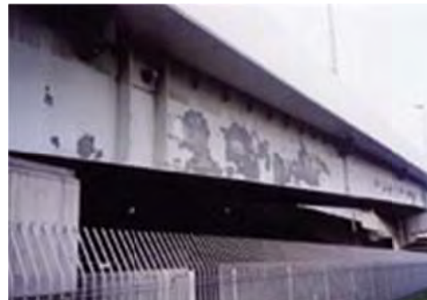
No 6: Member Girder
