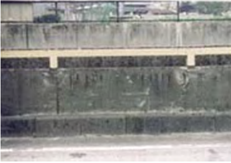
No 1: Member Railing wall
