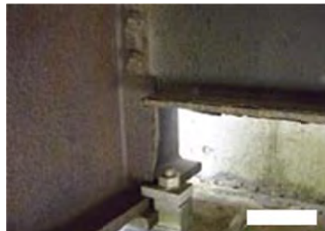
No 24: Member Cross beam
