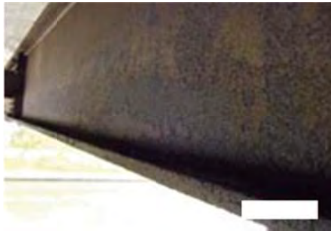
No 21: Member Girder
