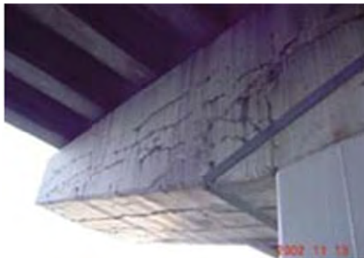
No 11: Membe Beam
