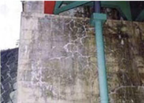
No 11: Member Abutment wall
