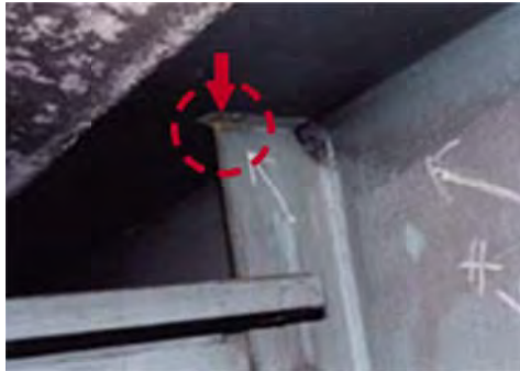
No 1: Member Girder
