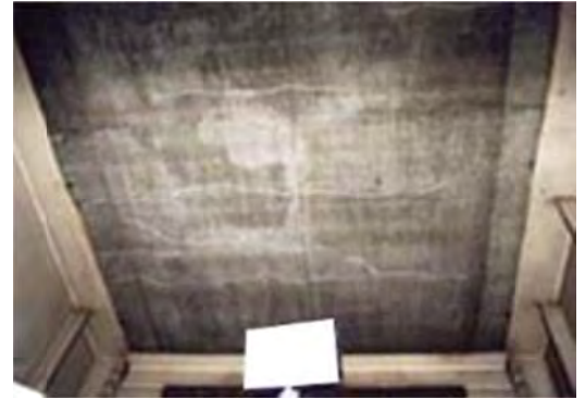
No 2: Member Floor deck
