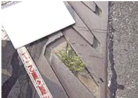
No 3: Member Expansion joint
