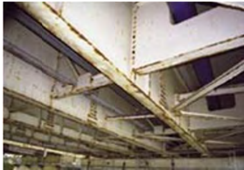
No 1: Member Girder
