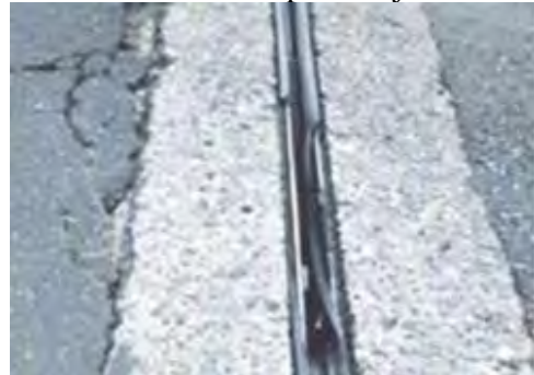
P 2: Member Expansion joint
