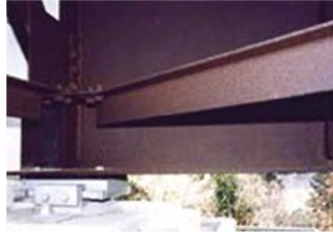
No 14: Member Lower bracing
