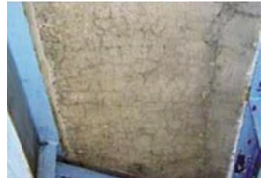
No 10: Member Floor deck
