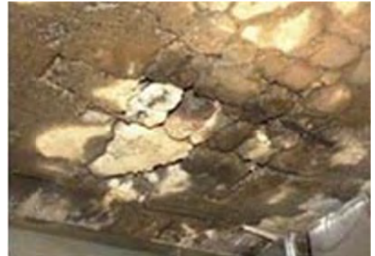
No 12: Member Floor deck
