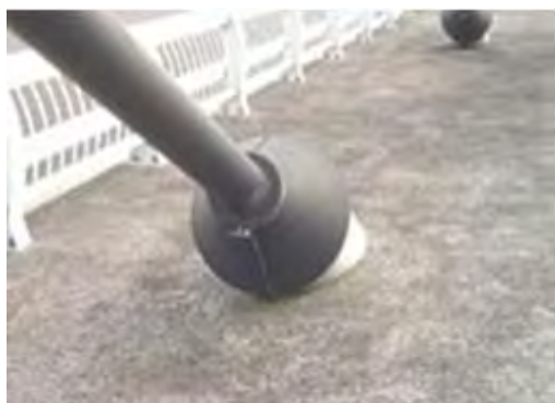
P18.3 Anchor of cable Stay Bridge (good)
