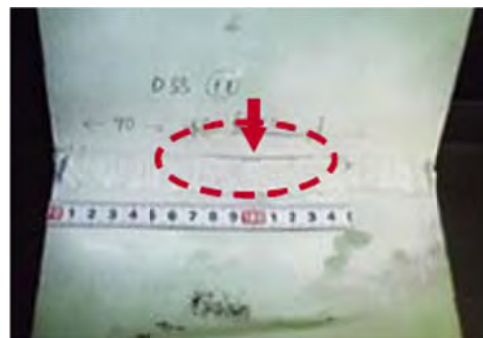
No 6: Member Cross beam
