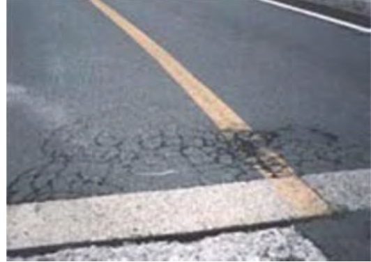
P 2: Member Pavement
