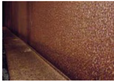
No 16: Member Cross beam
