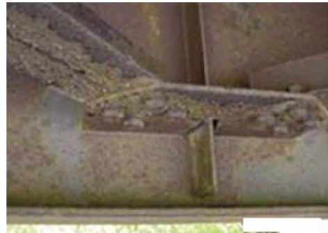
No 22: Member Lower bracing
