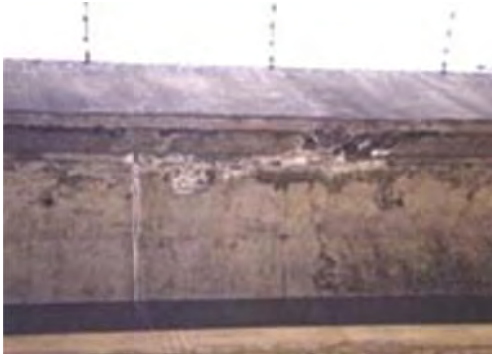
No 3: Member Floor deck
