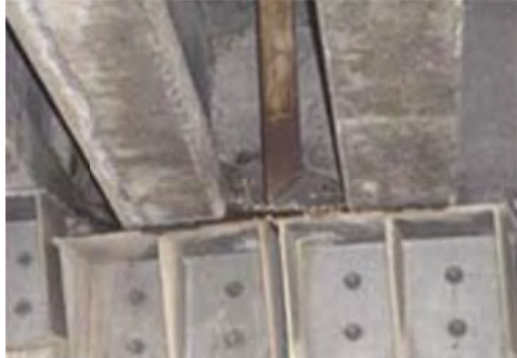
No 7: Member Bridge collapse prevention system
