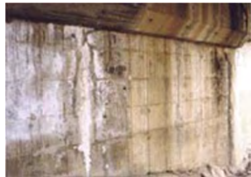
P8.4 Abutment wall
