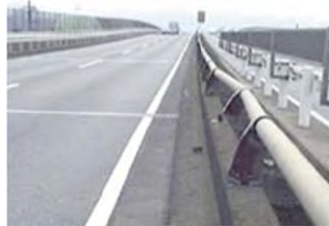
No 2: Member Railing
