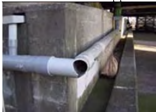
P 5: Member Drain pipe
