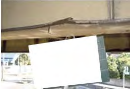
P 1: Member Girder
