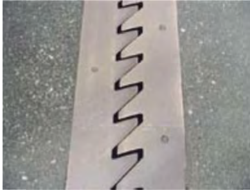
P 1 Member Expansion joint
