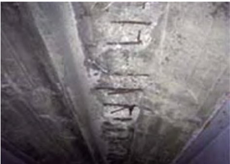
No 5: Member Girder
