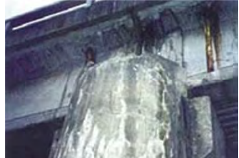
No 6: Member - Pylon wall
