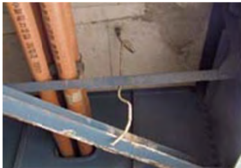
No 15: Member Lower bracing
