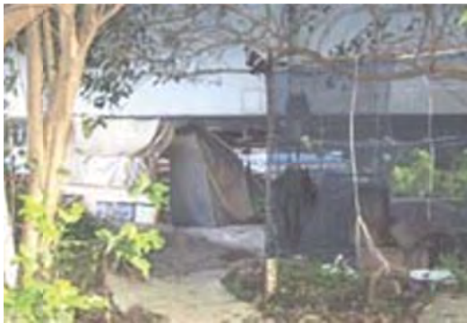
H17.3 Illegal usage
