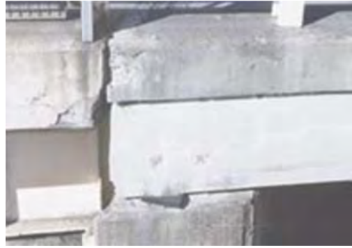
P 2 Member Girder
