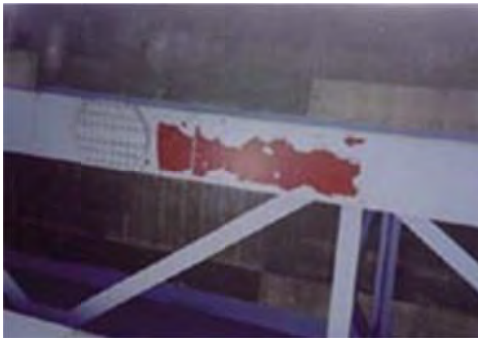
No 3: Member Girder
