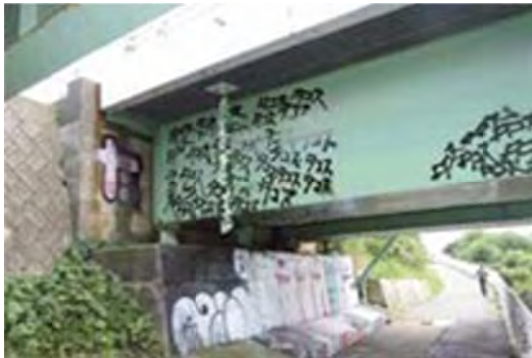
P3: Member Girder
