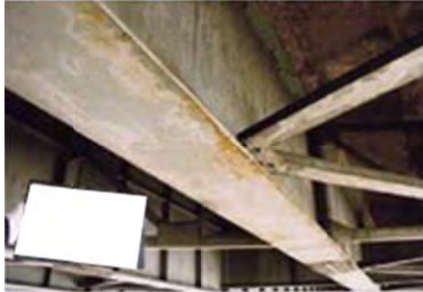
No 1: Member Girder
