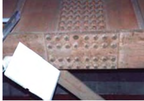
No 2: Member Girder
