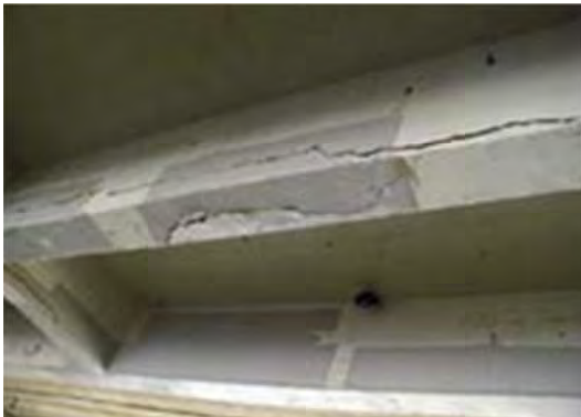
No 9: Member Girder
