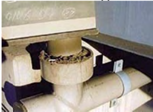
P3: Member Drain pipe
