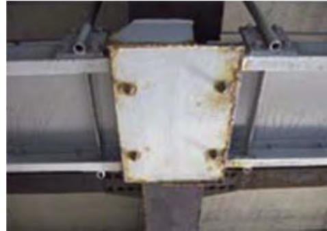
No 8: Member Inspection device
