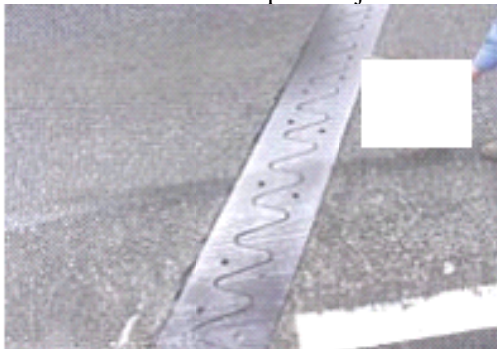
P 5 Member Expansion joint
