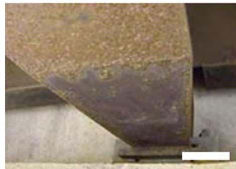
No 12: Member Girder
