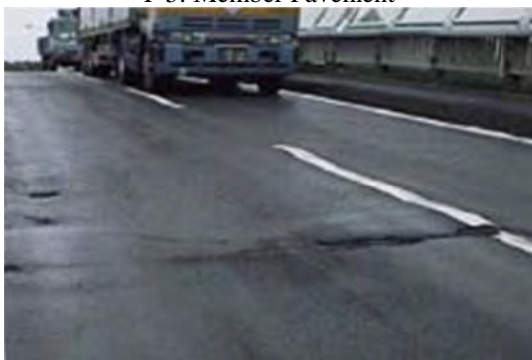
P 5: Member Pavement
