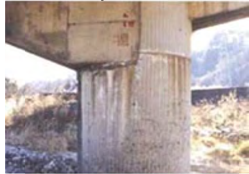
No 10: Member Pylon wall
