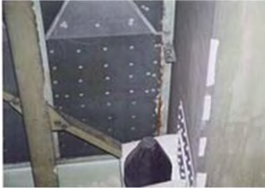
No 1: Member Floor deck
