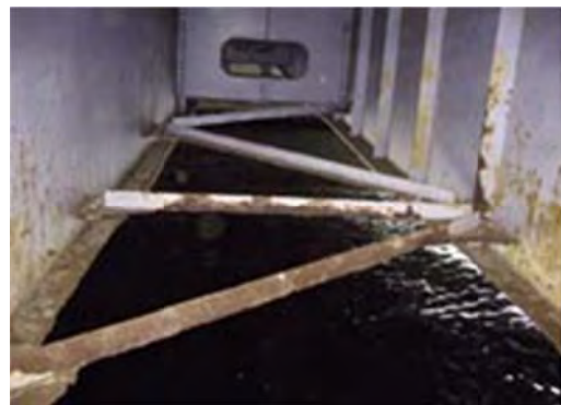
No 10: Member Lower bracing
