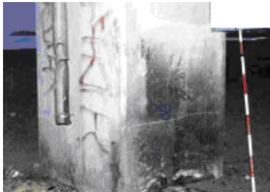
P5: Member Pier surface
