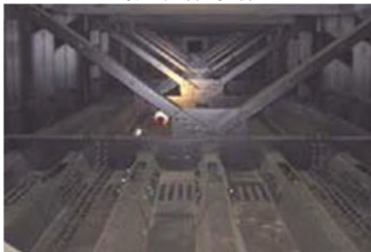
P5: Member Girder
