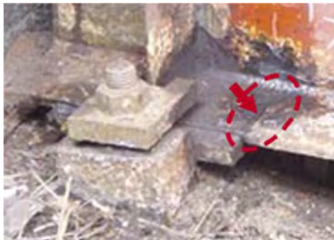
No 3: Member Girder
