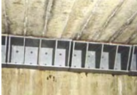
No 7: Member Bridge prevent collapse system
