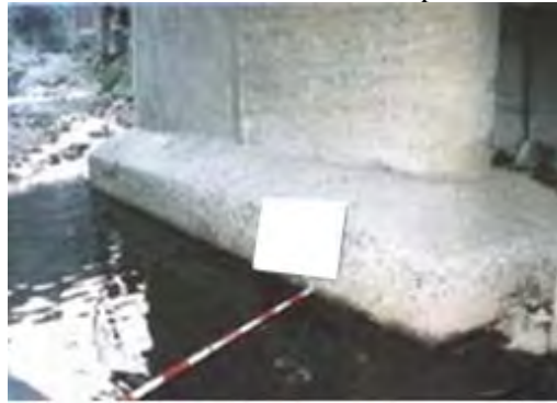
P 4: Member Base of pier
