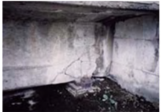
No 10: Member Girder
