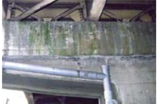
P8: Member Girder
