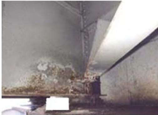
No 7: Member Girder
