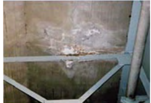
No 8: Member Floor deck
