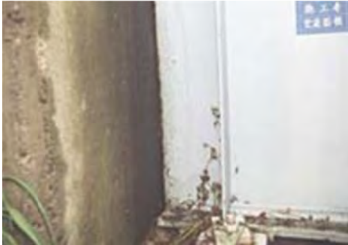
P 1 Member Girder
