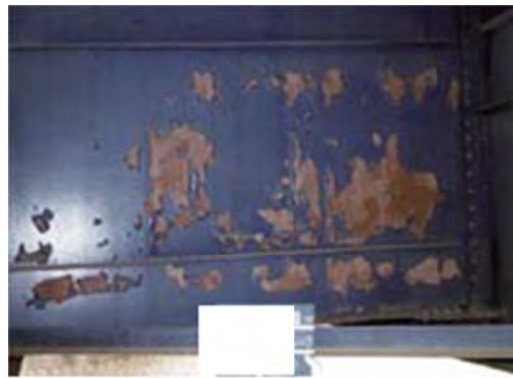
No 4: Member Girder
