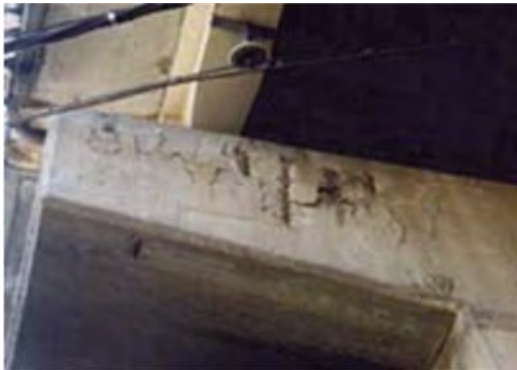
No 7: Member Pier beam
