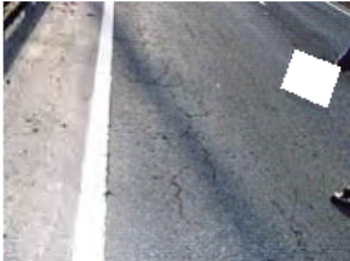
P 1: Member Pavement
