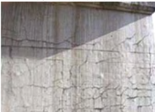
No 3: Member Abutment wall
