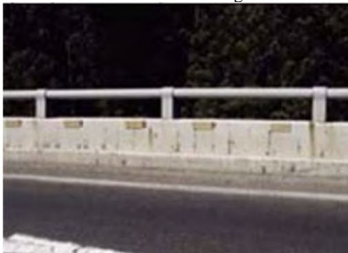
No 1: Member Railing wall
