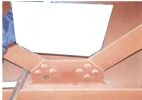
No 6: Member Lower bracing
