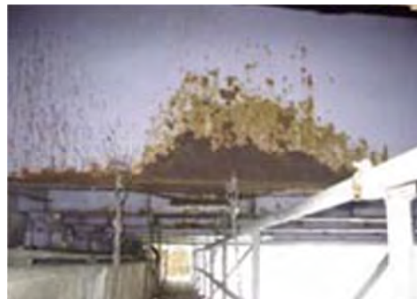
No 12: Member Girder
