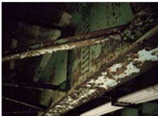
No 9: Member Girder
