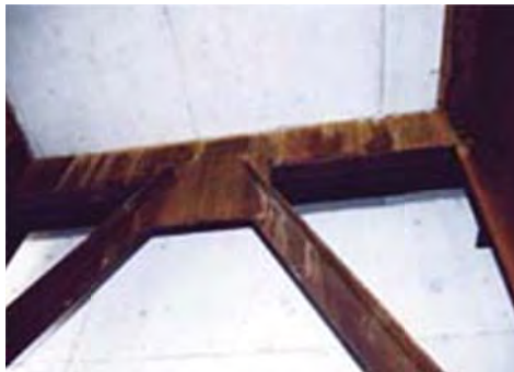
No 9: Member Diagonal bracing
