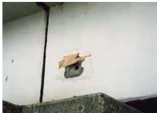
P 4: Member Girder
