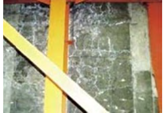
No 8: Member Floor deck
