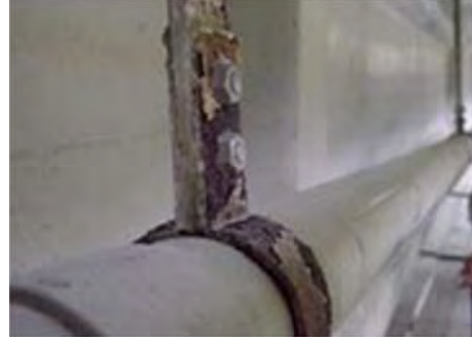
No 20: Member Drain pipe
