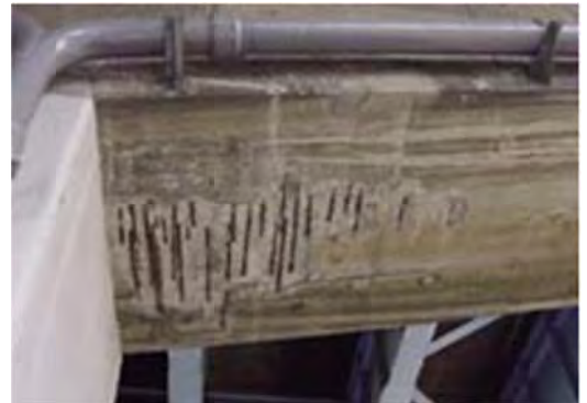
No 8: Member Pier beam
