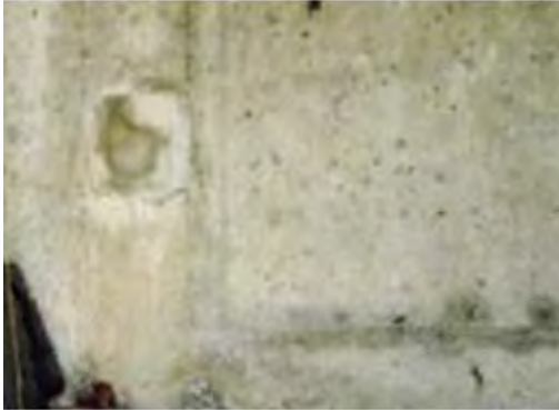
P 1: Member Girder
