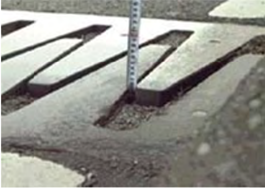
P 1 Member Expansion joint
