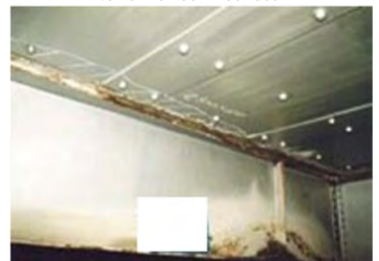
No 4: Member Floor deck
