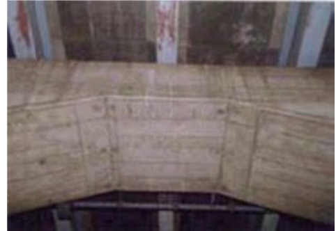
No 2: Member – Pier beam
