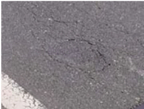
P 5: Member Pavement
