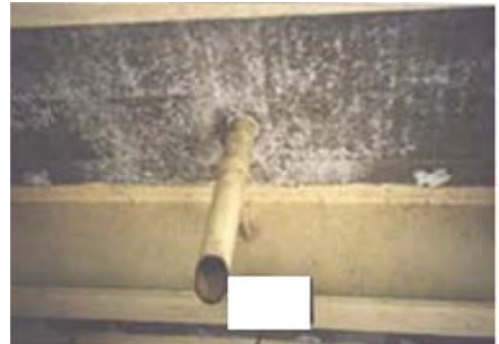
No 6: Member Floor deck
