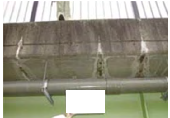
No 6: Member Floor deck
