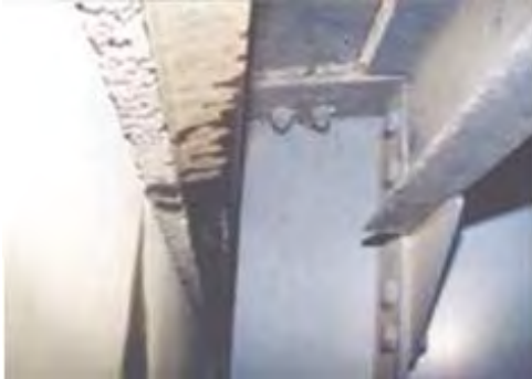
P 1: Member Expansion joint
