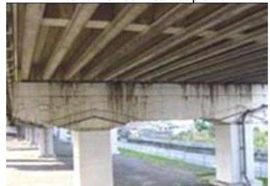
No 4: Member Beam at pier
