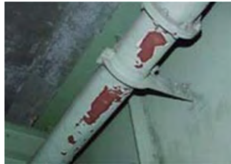
No 4: Member Drain pipe
