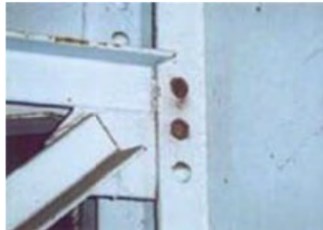
No 4: Member Cross beam
