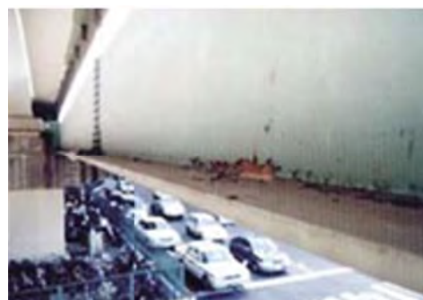
No 6: Member Girder
