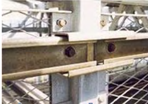
No 19: Member Inspection Facility
