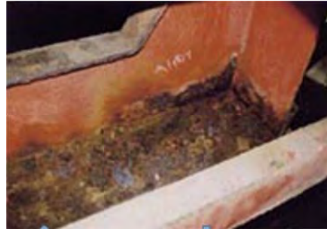
No 2: Member Girder
