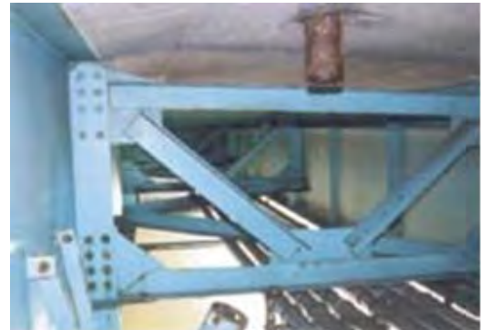
P20.11 Rapture at drain pipe
