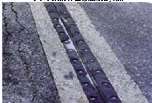
P 6: Member Expansion joint
