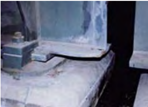
P 5: Member Girder
