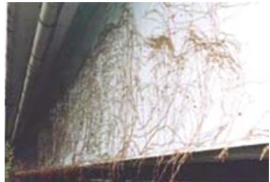
P6: Member Girder
