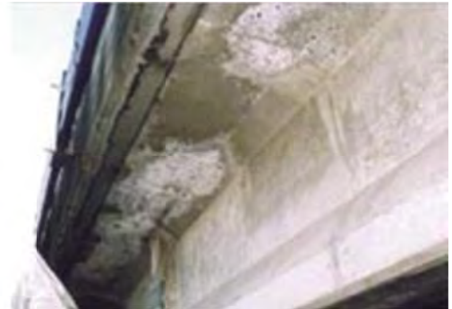
No 2: Member Floor deck
