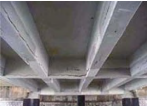
No 5: Member – Girder
