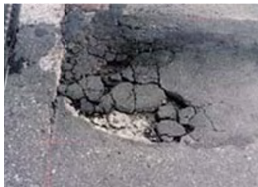
P 15.2 Digging of pavement
