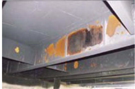
P2: Member Girder
