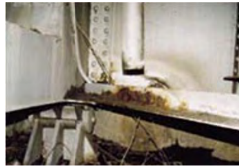
No 16: Member Lower bracing
