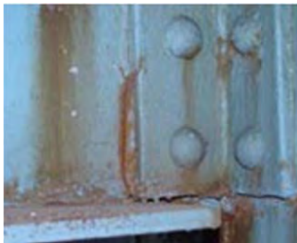
No 3: Member Cross beam
