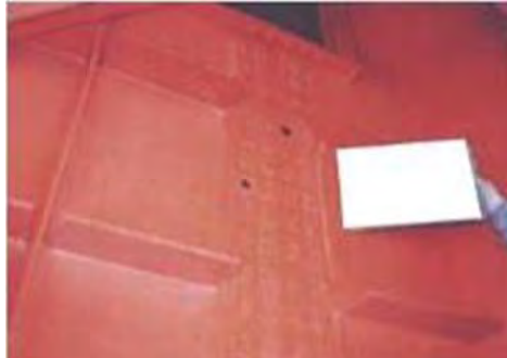
No 1: Member Cross beam
