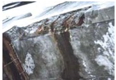
No 6: Member Floor deck
