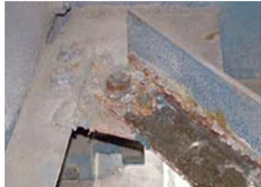
No 8: Member Lower bracing
