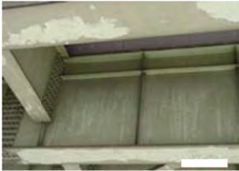
No 1: Member Girder
