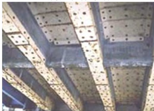
No 3: Member Girder
