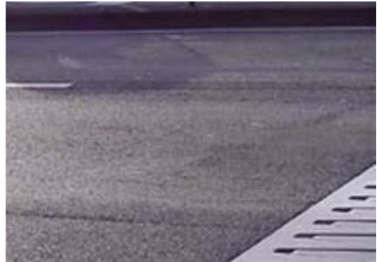
P 2: Member Pavement
