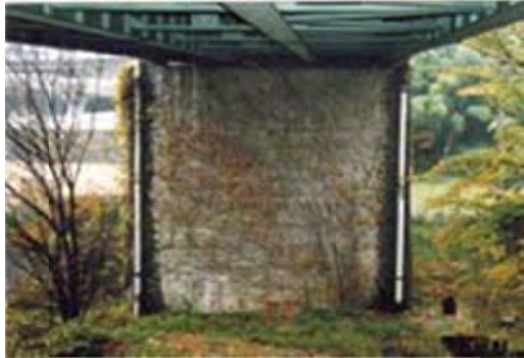
P9: Member Pier surface
