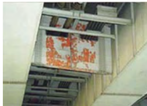
No 4: Member Cross beam
