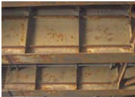
No 11: Member Girder
