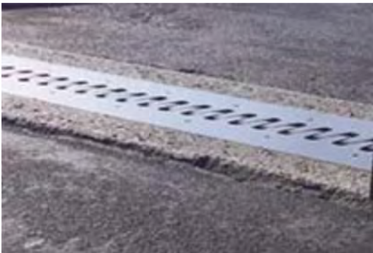
P 5: Member Pavement
