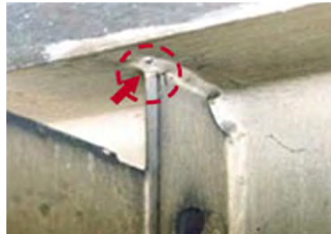
No 2: Member Girder
