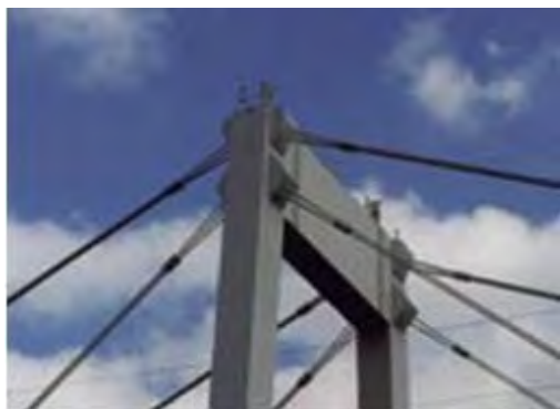
P18.5 Anchor of cable Stay Bridge (good)
