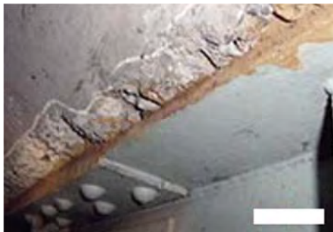
No 5: Member Girder
