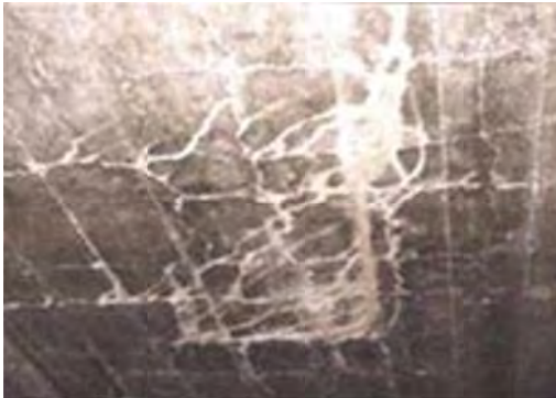
No 11: Member Floor deck
