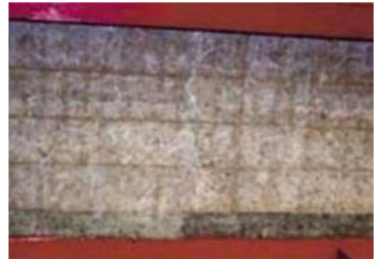
No 4: Member Floor deck
