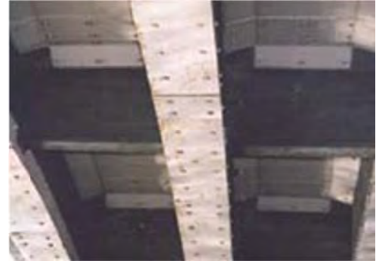
No 2: Member Girder
