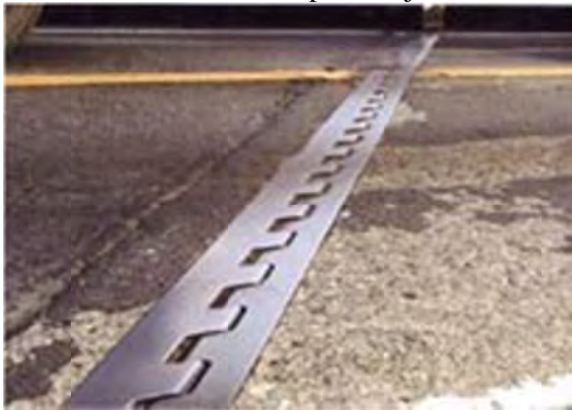
P 3: Member Expansion joint
