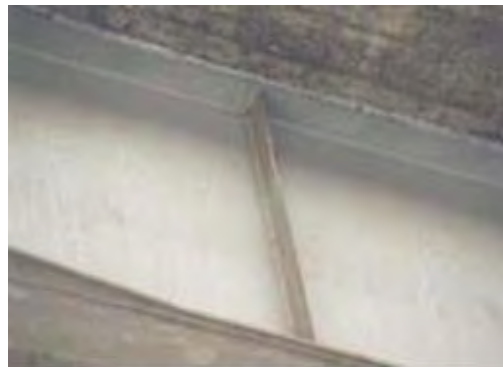
P 6: Member Girder
