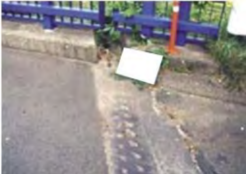
P 5: Member Expansion joint
