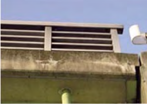
No 1: Member - Floor deck
