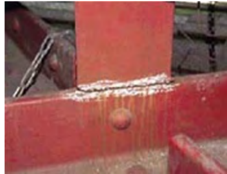
No 2: Member Lower bracing
