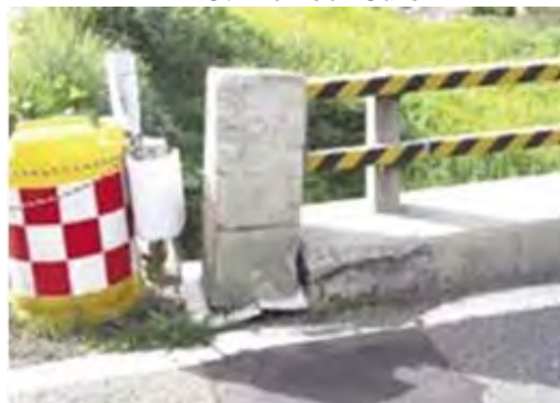
P 3: Member Curb
