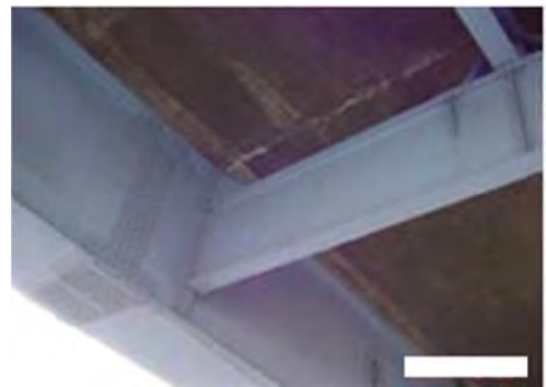
No 4: Member Floor deck
