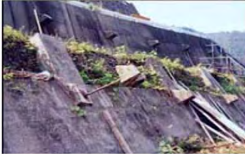
Photo 3.1 Ground anchor ship
