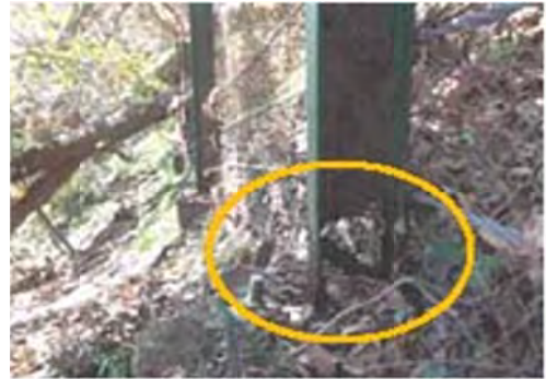
Photo 5.6 Steel member corrosion (rock fall prevention H beam base)
