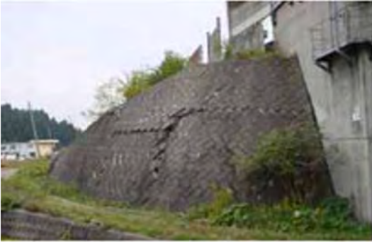
Photo 4.1 Wall crack
