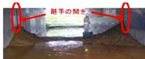
Photo 7.11 Flow of water and sediment or joint opening
