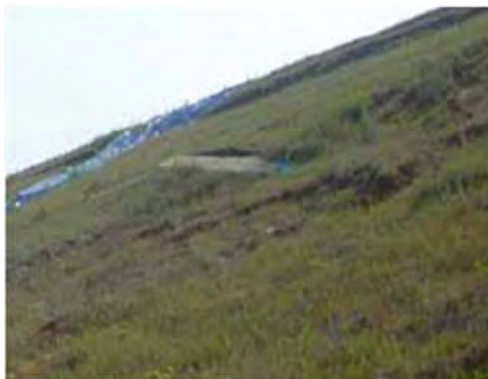
Photo 2.1 Whole slope failure
