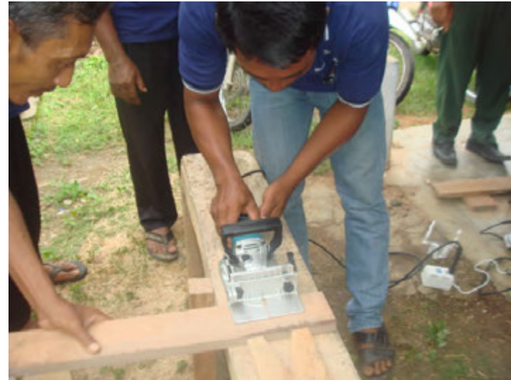
Making a hole by joint cutter
