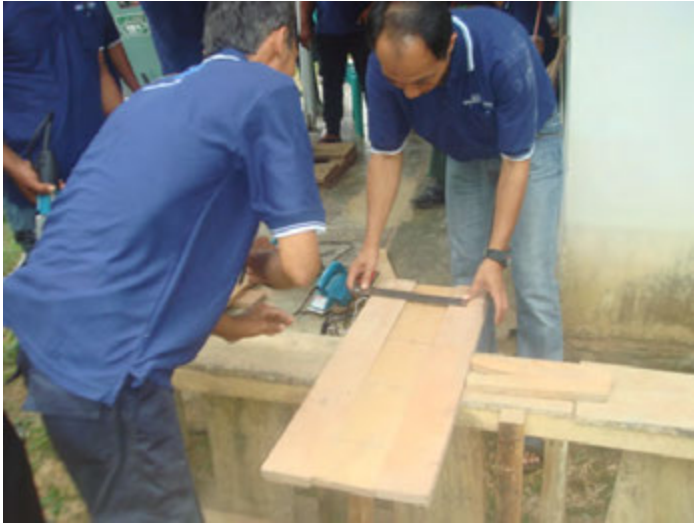
Adjusting three boards
