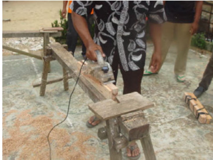
Making a hole by joint cutter
