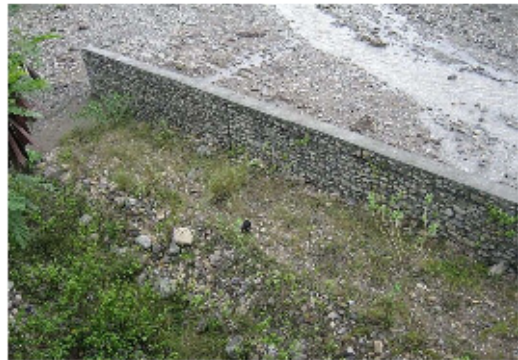
Fig. 2.2.23 Revetment Condition on Left Bank Side of Mola Bridge
