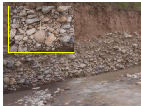
Fig. 2.2.16 Existing gravel and deposition layer at riverside
