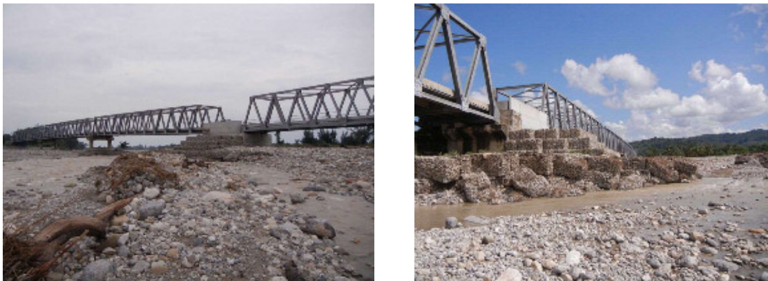
Photo 2.2.18 Current Situation of Bridge Pier Provided with Protection Work
