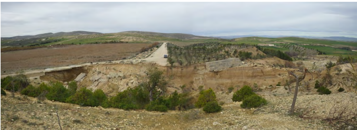
General view from the right side of dam, SI-6 Zaaroura
