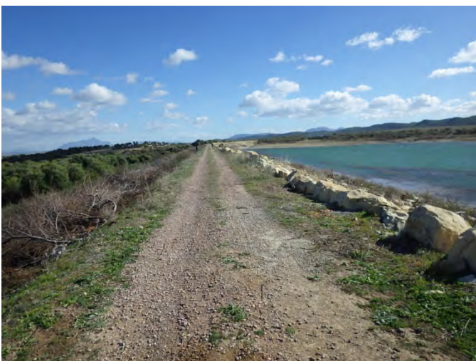
Dam crest and reservoir, ZA-3 Enfidha
