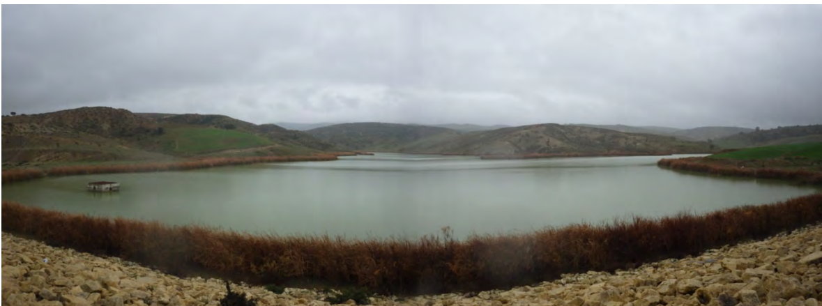
General view of reservoir, BE-3 Slougua
