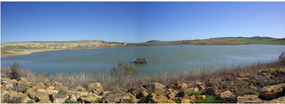
General view of reservoir, BE-5 Sidi Yahia
