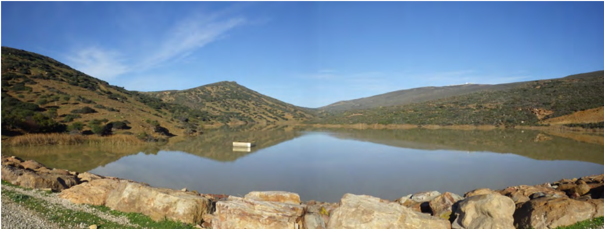
General view of reservoir, NA-1 Tabouda
