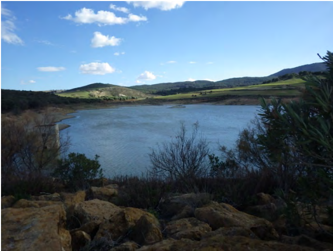
View of reservoir from left side, ZA-4 Guissat
