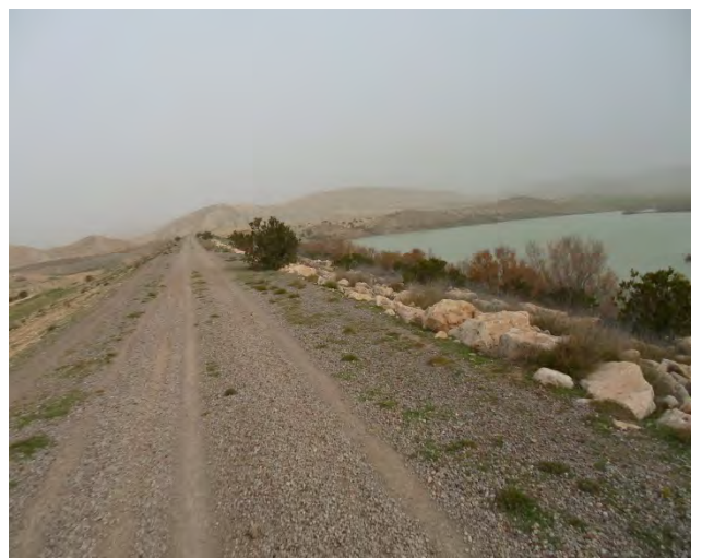
Dam crest and reservoir, KE-2 Rouijel
