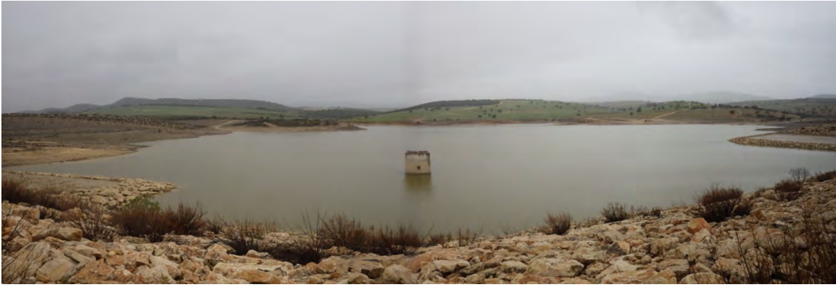
General view of reservoir, BE-4 Kashbar
