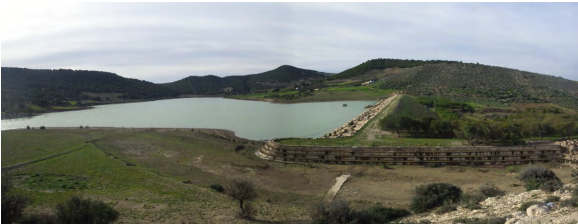
General view from right side of dam, SI-8 Ain Shigaga
