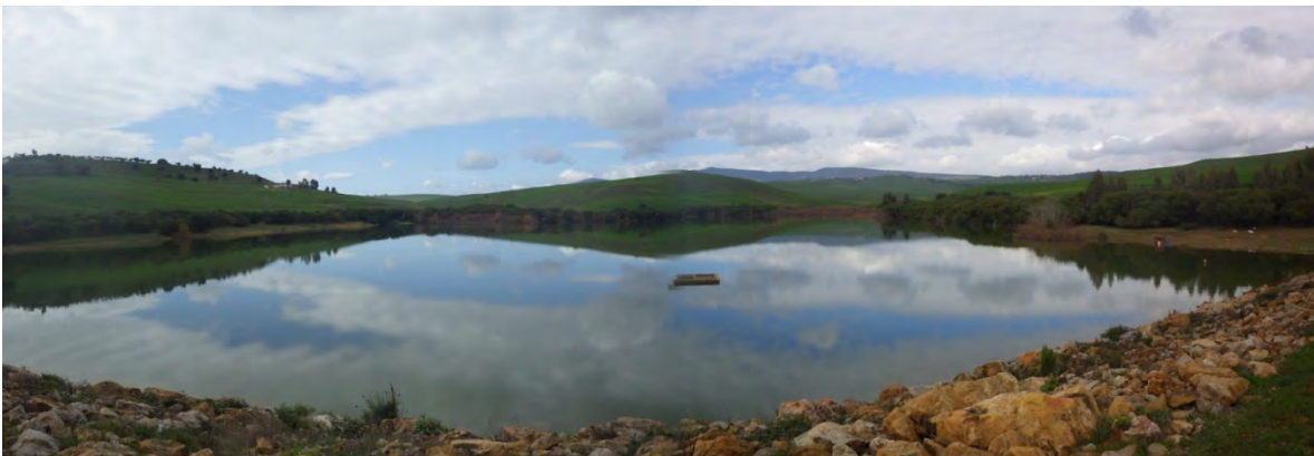
General view of reservoir, JE-1 Sammar
