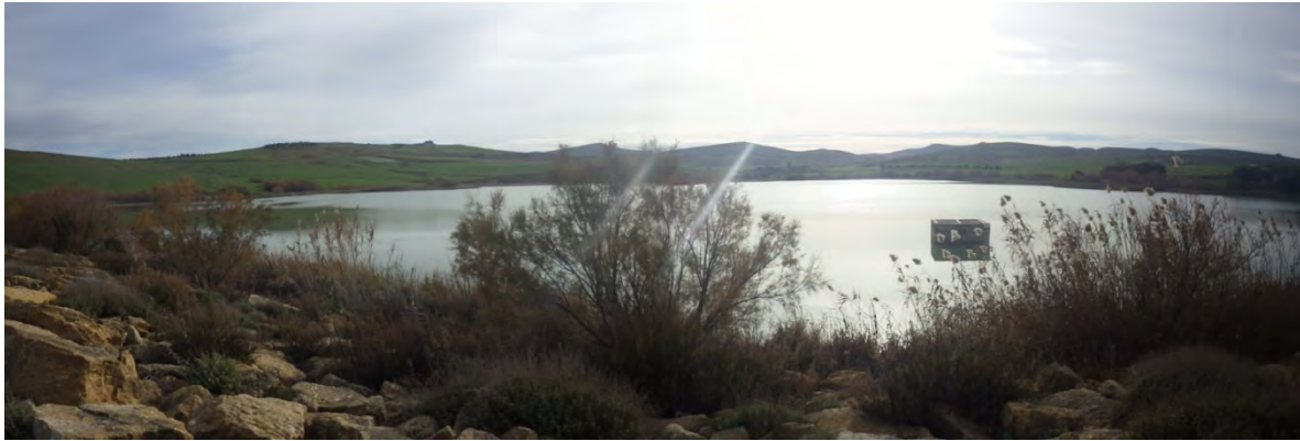
General view of reservoir, SI-2 Mechaiker
