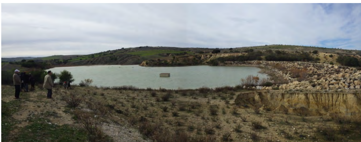
General view of reservoir and upstream of dam, SI-4 Meskaya
