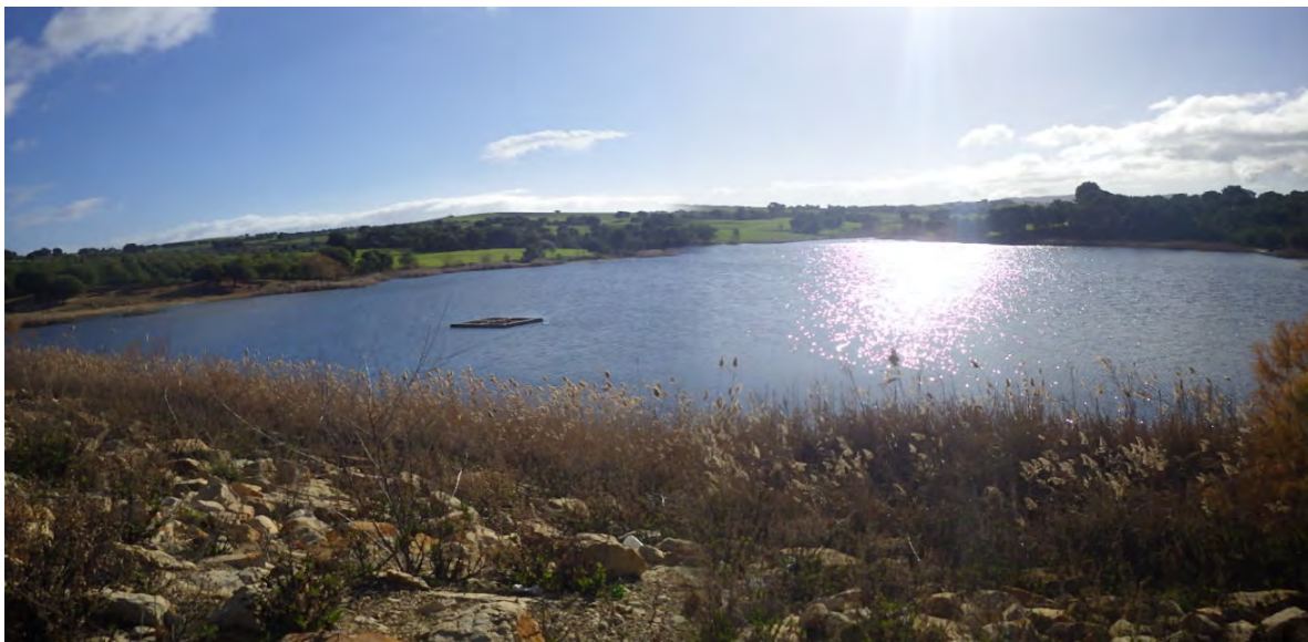
General view of reservoir, SI-3 Nchem
