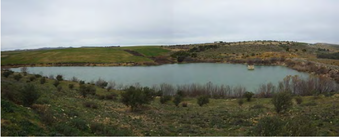
General view of reservoir, SI-10 Joura
