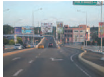
Ramp for left-turning vehicles on the Mactan Island side of the Second Mactan Bridge
