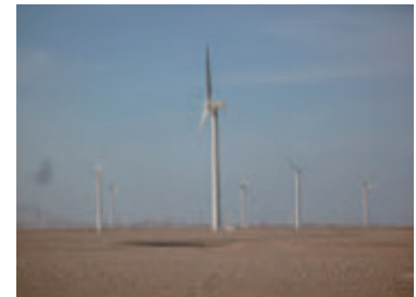
Wind power plant constructed in this project
