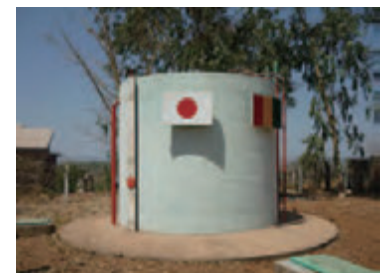
Water tank of piped water supply facility
