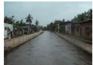
Drainage system after the implementation of the project
