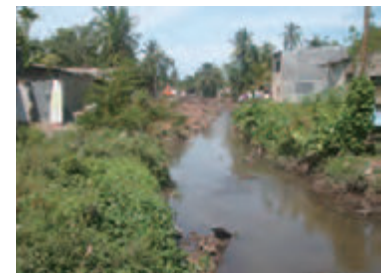
Drainage system prior to the implementation of the project (taken in 2002)
