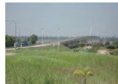
Second Mekong International Bridge: SMIB (taken from Lao side)
