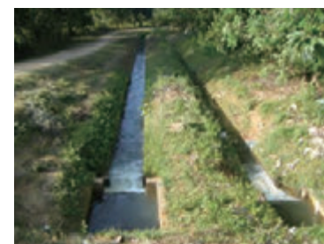
Dual Canal System: The left is for rice and the right is for other crops
