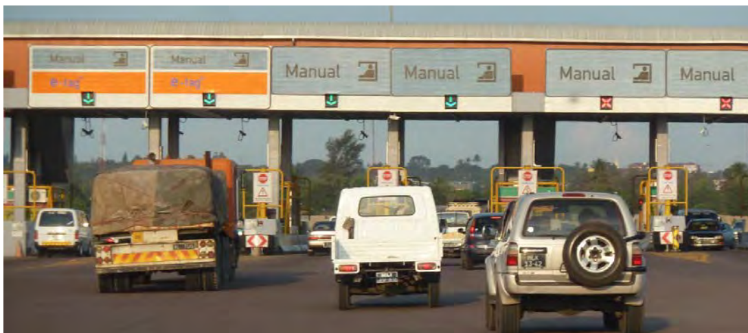
The N4 Toll Gate
