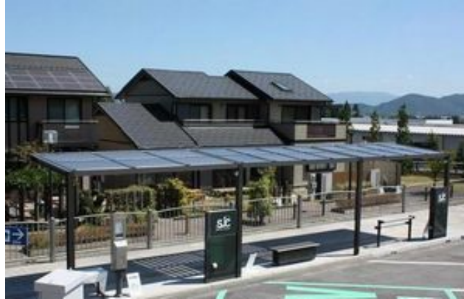
Figure 12.1: Bus Station with PV Panel
