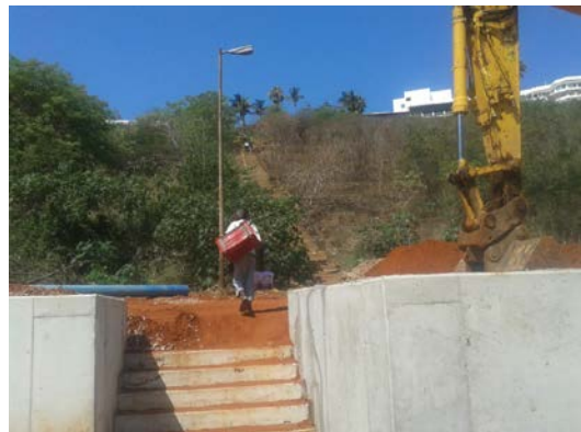
Source: JICA Project Team
