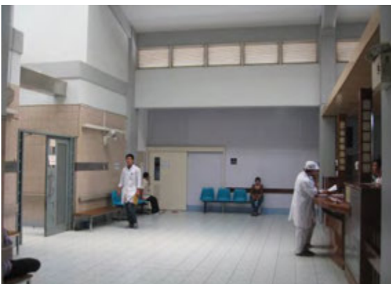
Wall installed to renovate NCU-B on the second floor of the North Building
