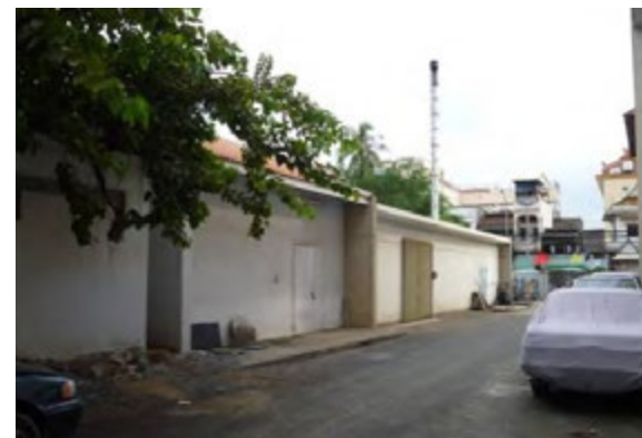
G: Incinerator/storehouse modified by Japan's technical assistance in 2001
