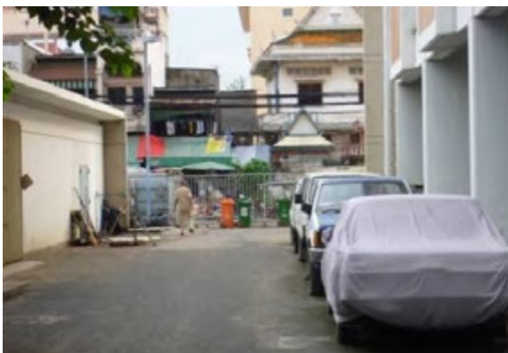
F: Garbage truck gate constructed with the hospital's
