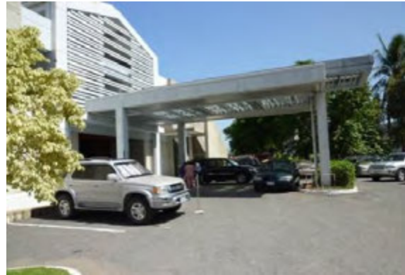
B: Main access to Outpatient Service Department
