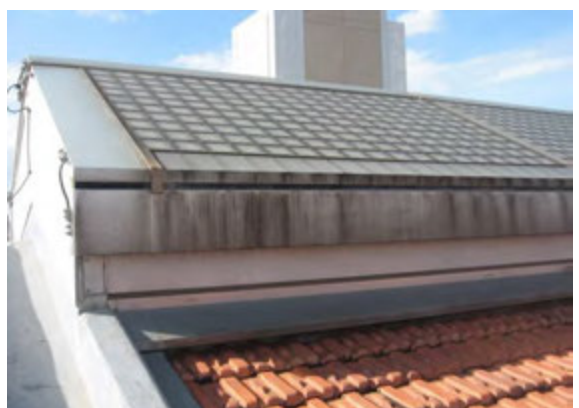
Glass block skylight
