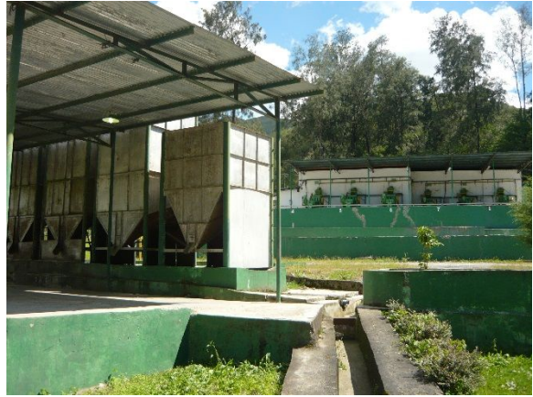
CCT (Coffee factory)
