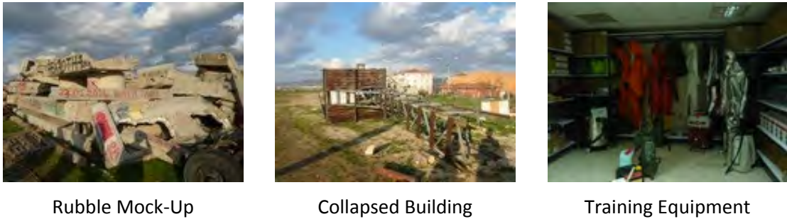
Figure 3.3.9 AFAD Bursa Training Facility
