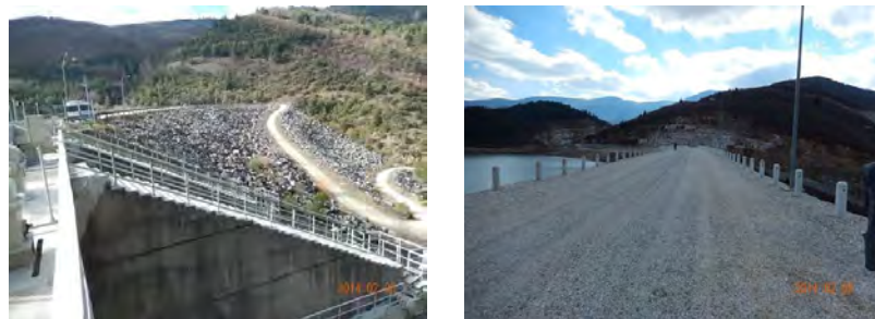
Doganci Dam Nilufer Dam
