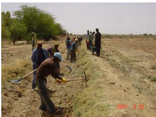
Repairing work of existing canal done by farmers' participation. March, 2011 (Podor, Donaye IT4 area)
