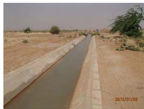
Lining work of main canal. January, 2013 (Podor, Ngane area)
