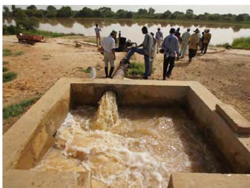
Water pumping to the division box. September, 2011 (Podor, Diatar2 area)
