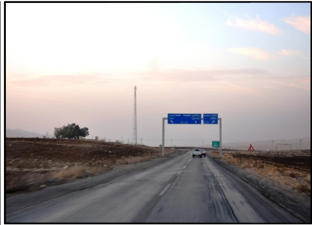
Figure 5.4.8 Main road near Gomaspan SS (Arrow 6 in Figure 5.4.2)
