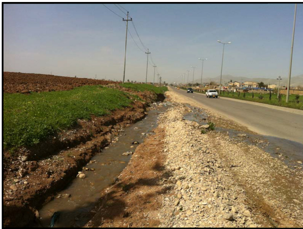
Figure 5.4.15 Main road near Arbat SS (Arrow 5 in Figure 5.4.9)
