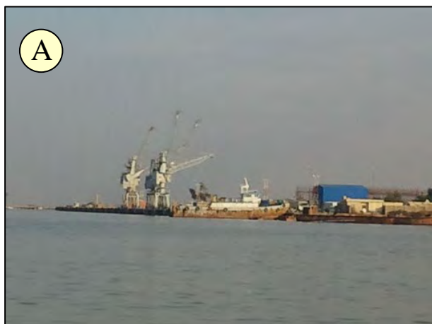
Figure A6. 11 (Basra) Loading Facilities of Port of Abu Flus
