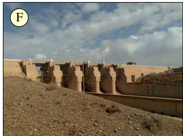
Figure A3. 15 (Diyala) Hemren Dam 5 Gate
