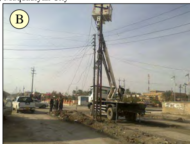
Figure A3. 10 (Diyala) Repair of Electricity
