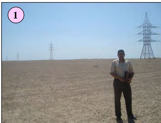
Figure A2. 4 (Al-Anbar) 400kV Transmission Line
