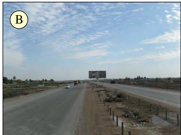
Figure A7. 5 (Al-Radwaniyah) Highway
