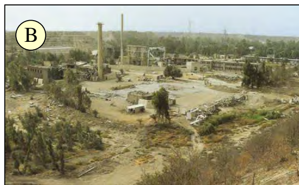
Figure A8. 8 (Al-Madaain) Nuclear Plant under Construction
