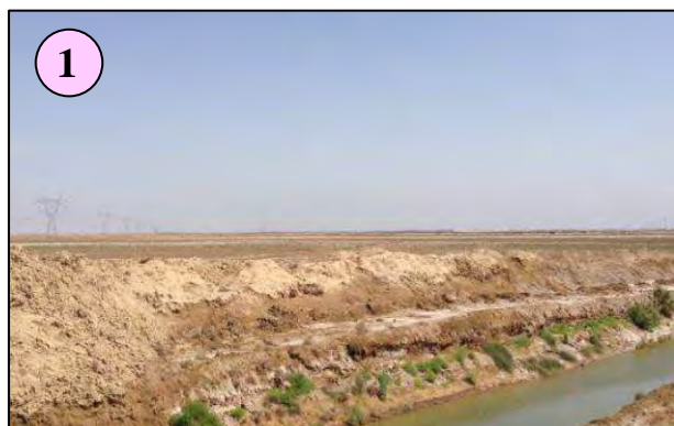
Figure A5. 3 (Missan) 400 kV TL Line and Cannel
