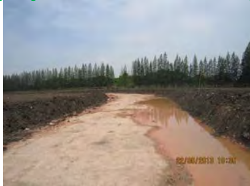
After project: Construction stage
