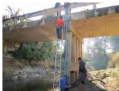
Installing water level gauge
