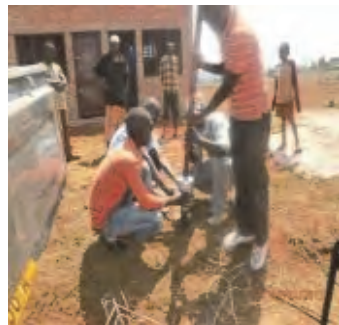
Cutting metal pipe
