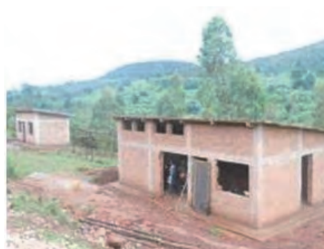
Seed Storage Under Construction
