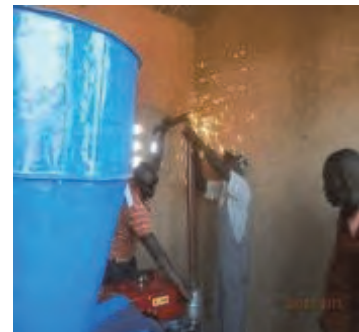
Weld two pipes
