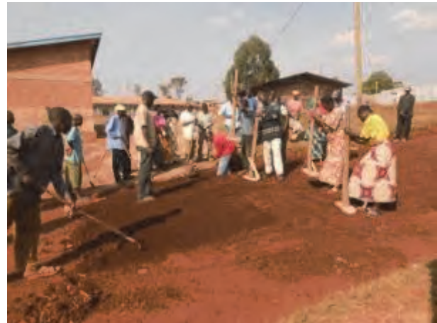
Practical workshop for maintenance training
