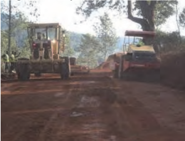
Construction works with grader and roller
