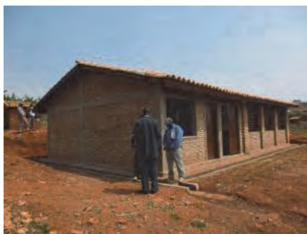
Building for carpentry works of PP8
