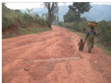
Fragile condition of the road between Bukirasazi and Buraza
