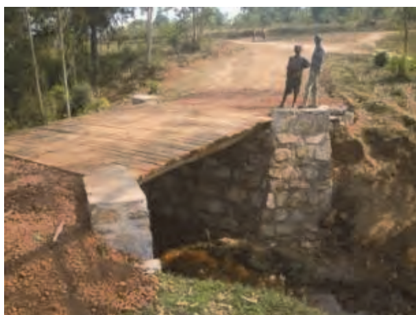
Constructed bridge of PP7
