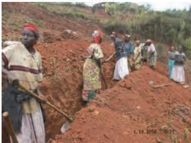
Making contour lines for grass fixing
