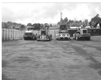
Base of contractors
