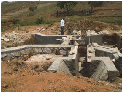
Intake 2 under construction
