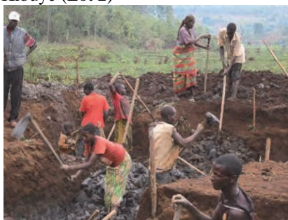
People are working at Intake 1
