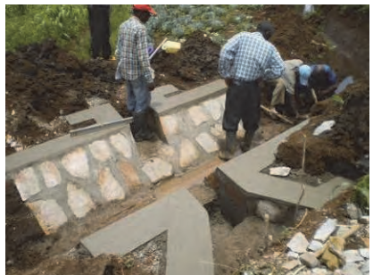
Spillway to be finished
