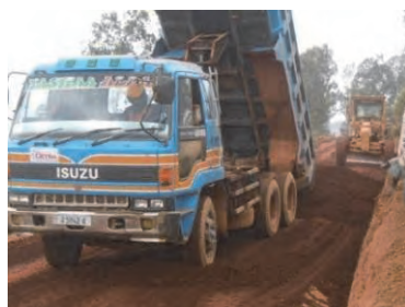
Placing the Laterite
