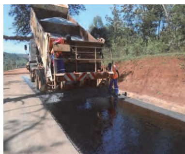
Spreading of bitumen and granulates
