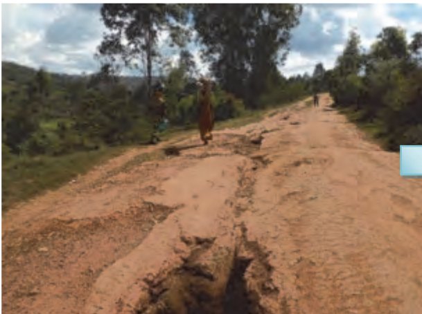
(Before) the road rehabilitation
