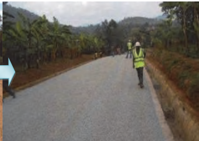
(After) the road rehabilitation
