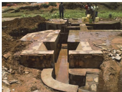
Intake 2 under construction
