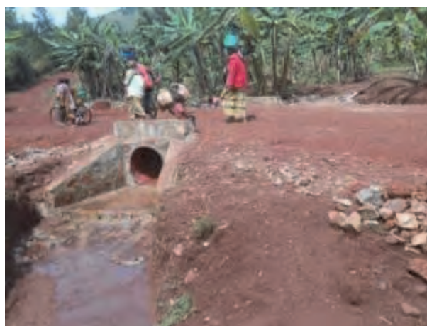
Constructed culvert of PP7
