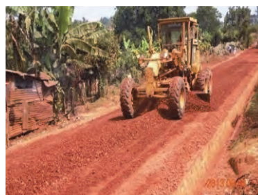
Spreading the Laterite
