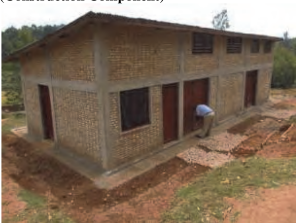
Multipurpose shed of PP1
