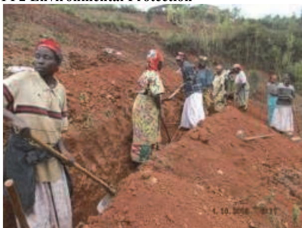
Making contour lines for grass fixing
