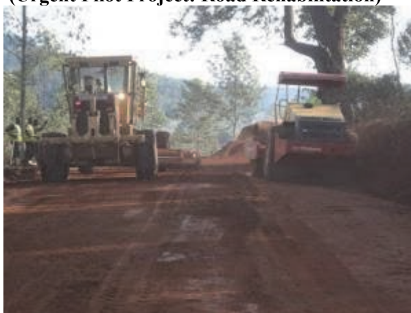
Construction works with grader and roller
