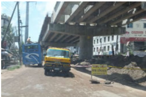
Overpass Construction by CDA
