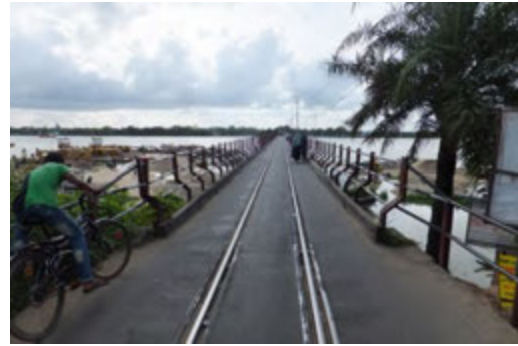
Kalurghat Bridge Deck
