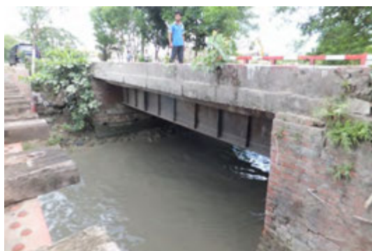
Bridge on Airport Road (1)
