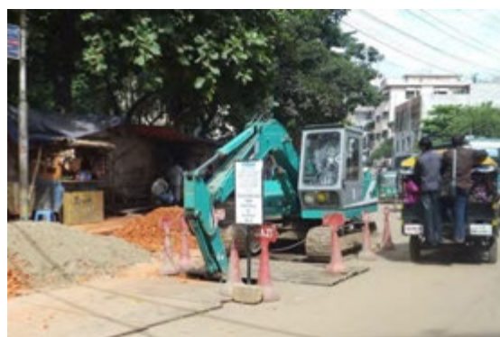
Pipe Installation in the City (2)
