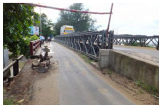
Bridge on Airport Road (2)
