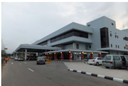
Airport Terminal Building
