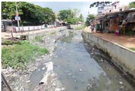
Retaining Wall of Mehesh Kali khal
