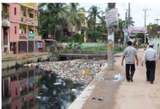
Garbage Stagnating at Chaktai Khal
