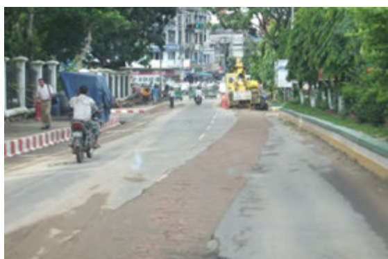
Pipe Installation in the City (1)
