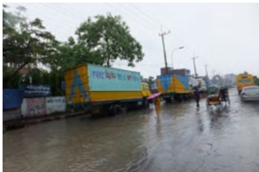
Flooding on Port Connecting Road
