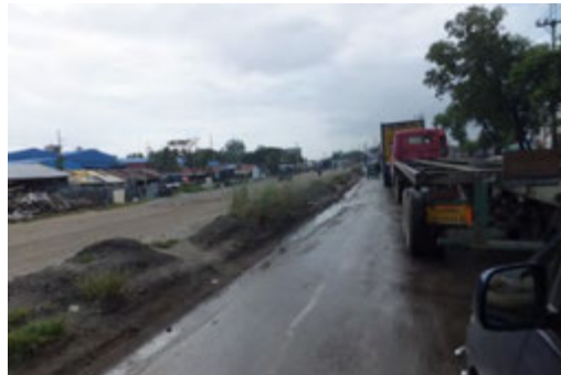
On-going Highway Widening
