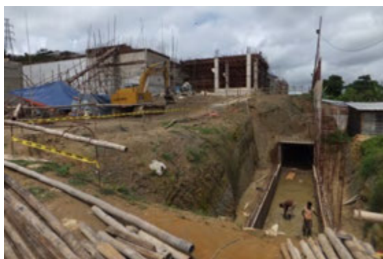
Reservoir Construction Site
