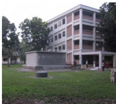
Figure 10-7: Typical Structure of School Cum Cyclone Shelter
