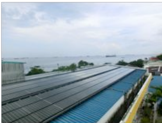
Figure 10: PV Modules at Thaajudeen School, Maldives
