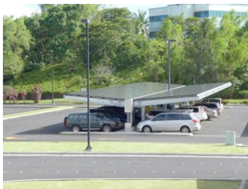
Figure 9: PV Modules at Palau International Airport
