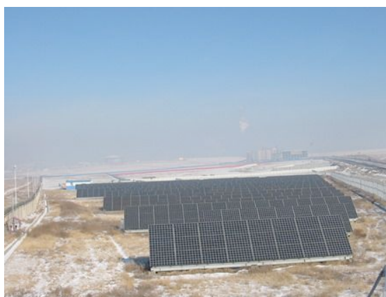
Figure 8: PV Modules at Chinggis Khaan International Airport, Mongolia
