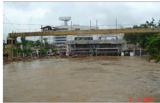
Flood in MANGGARAI GATE (2007)
