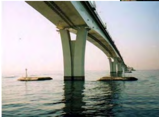
Steel Box Girder Bridge (Tokyo Bay Aqua Line) Span Length: 240 - 80 m 7
