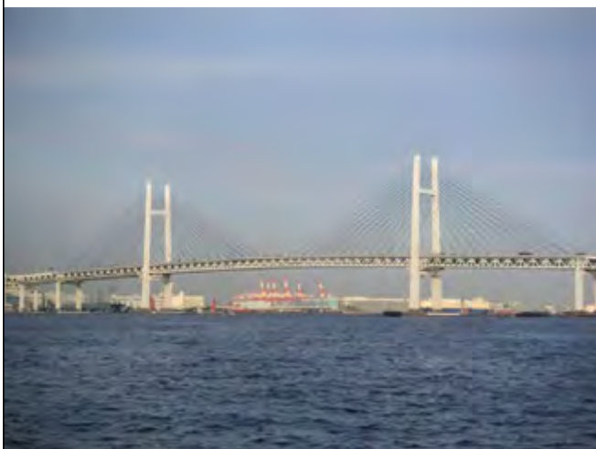
Steel Cable Stayed Bridge (Yokohama Bay Bridge) Span Length: 460 m
