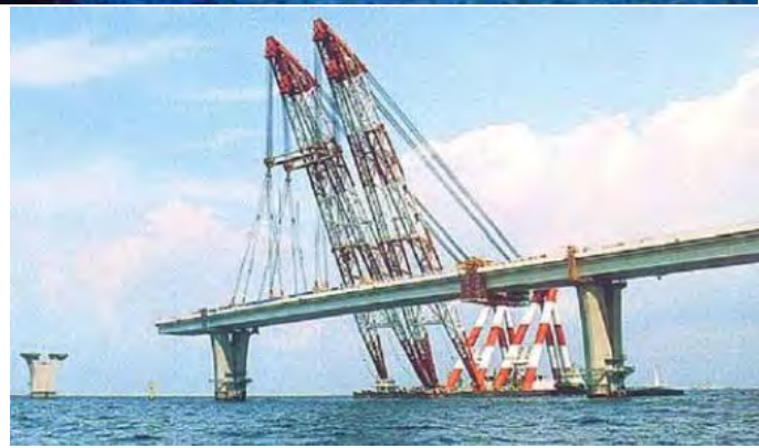
Steel Box Girder Bridge (Tokyo Bay Aqua Line) Span Length: 240 - 80 m 7
