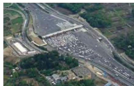
Before installation ETC
