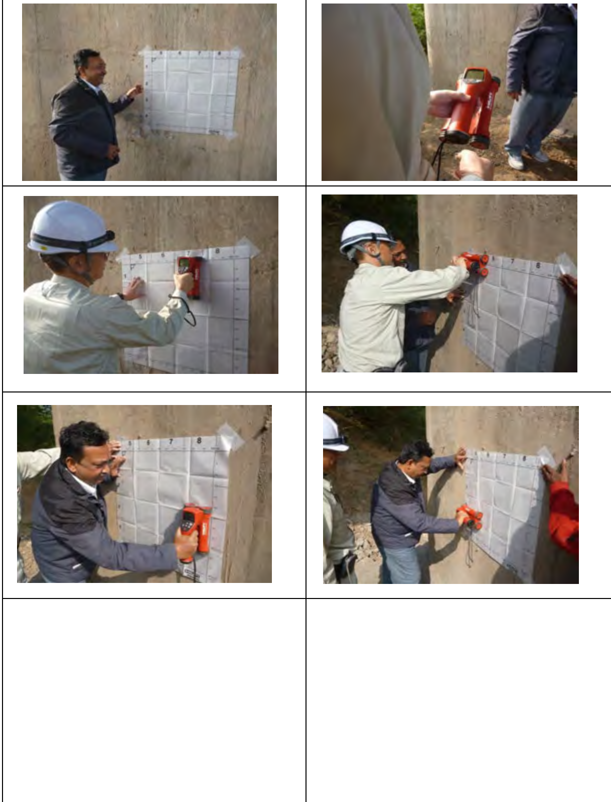
Photoes (Concrete cover survey: Electro magnetic redar)
