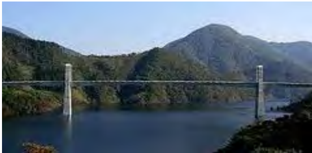
Tokunoyama Hattoku Bridge ( Span Length: 220 m)
