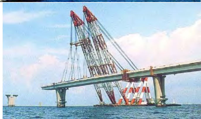
Steel Box Girder Bridge (Tokyo Bay Aqua Line) Span Length: 240 - 80 m
