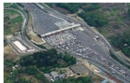
Before installation ETC
