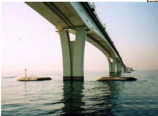
Steel Box Girder Bridge (Tokyo Bay Aqua Line) Span Length: 240 - 80 m
