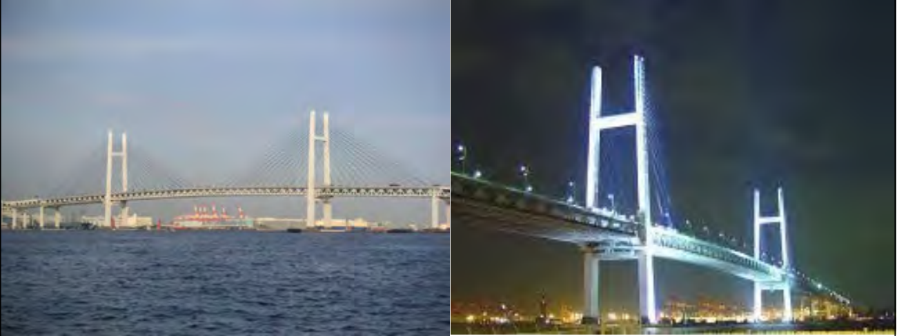
Steel Cable Stayed Bridge (Yokohama Bay Bridge) Span Length: 460 m
