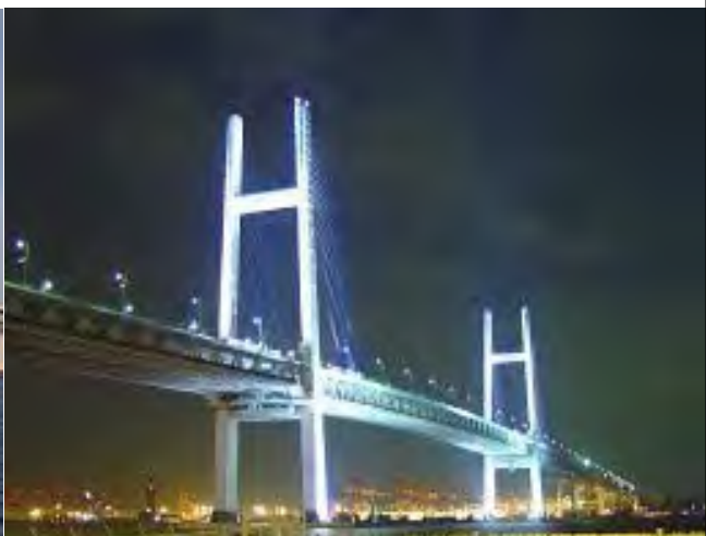
Steel Cable Stayed Bridge (Yokohama Bay Bridge) Span Length: 460 m
