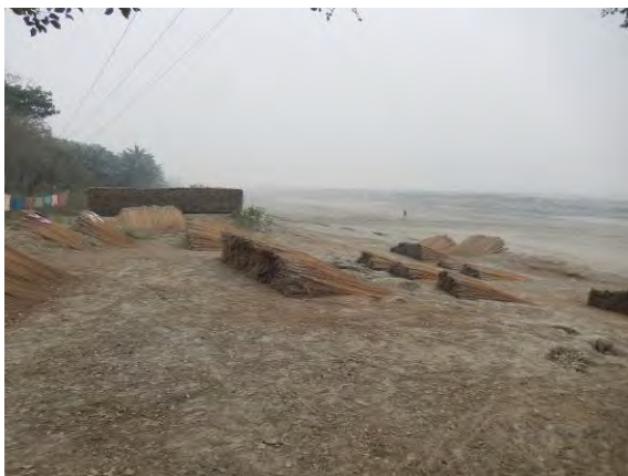
Dhuburi-Phulbari Bridge Candidate site (Assam side)
