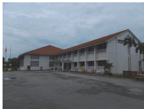
University building constructed by “Improvement of Facilities and Equipment of Faculty of Agriculture, Can Tho University”
