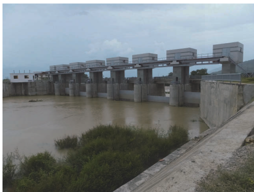
Headworks constructed at the beginning of the main canal of Phan Ri – Phan Thiet Irrigation Project.
