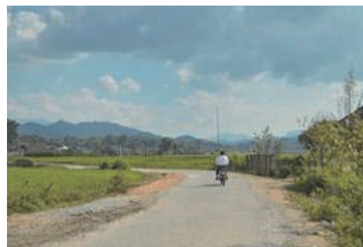
Project road after improvement
