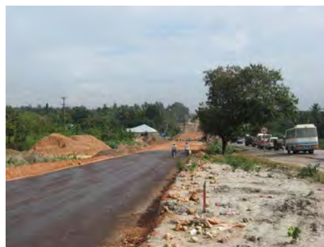
Photo 5.8: Bagamoyo Road Widening
