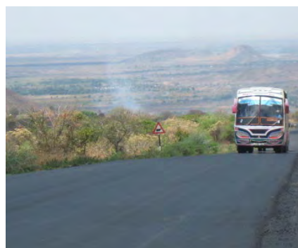
Photo 5.2: Newly Rehabilitated Section of T1
