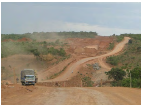
Photo 5.3: Tunduma-Ikana under Construction
