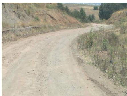
Photo 5.5: Gravel Road, T8
