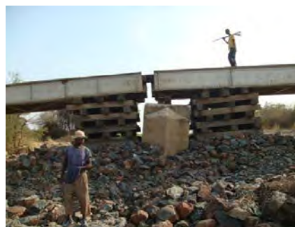
Photo 6.2: Bridge at Km 517, Damaged by Floodwaters
