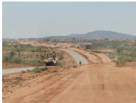
Photo 5.4: Laela-Sumbawanga under Construction
