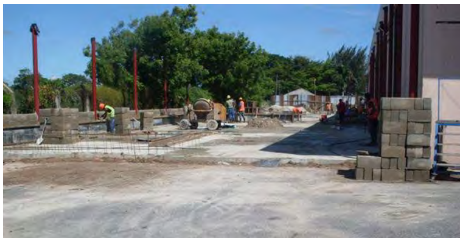
Photo 7.2: Construction of New Cold Room (Ground Floor Slab Concrete Works)
