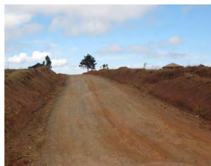
Photo 5.6: Typical Earth Road, T8
