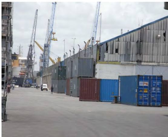
Photo 4.1: Scattered Containers in the Yard
