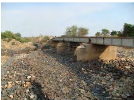
Photo 6.2: Bridge at Km 517, Damaged by Floodwaters
