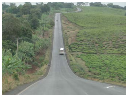
Photo 4.28: Steep Slope with Short Sight Distance
