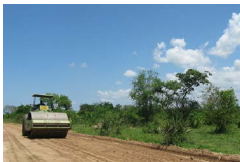
Photo 4.23: Compacting Earth Road by a Roller
