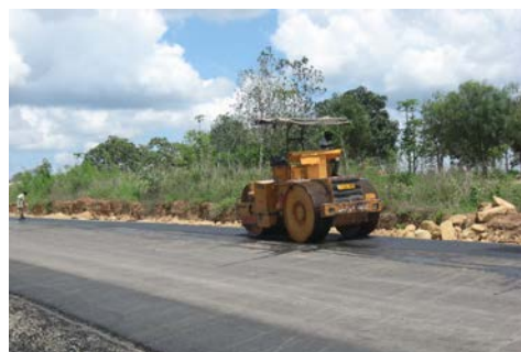
Photo 4.24: Upgrading to Bitumen Standard
