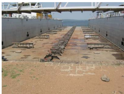
Photo 3.42: No.2 Floating Dock (New)
