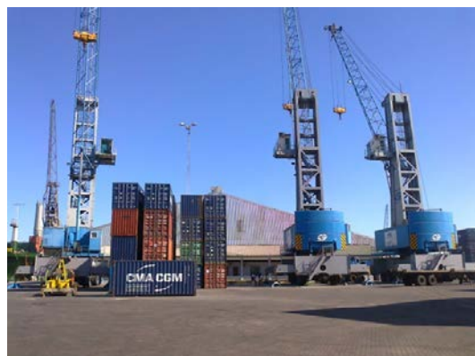
Photo 3.2: Mobile Harbour Cranes
