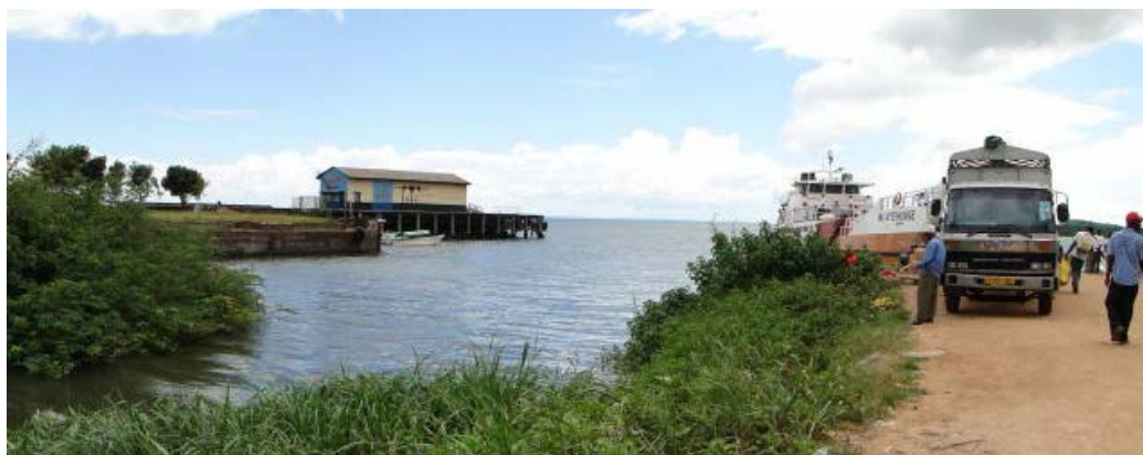
Photo 3.32: TPA Jetty and Private Jetty at Nansio
