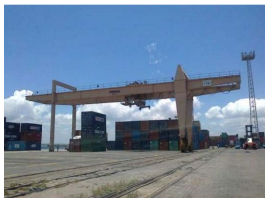
Photo 3.22: Rail Mounted Gantry Crane
