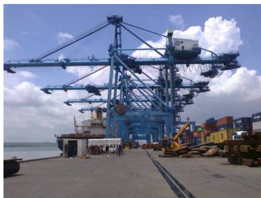
Photo 3.18: Ship-to-Shore Gantry Crane (4 Nos.)
