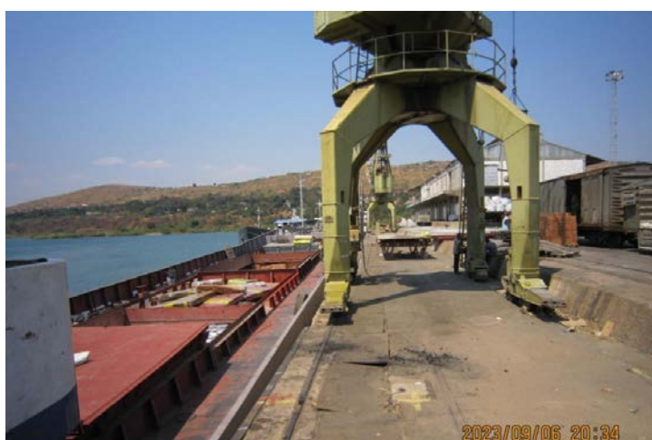
Photo 3.43: General Cargo Wharf at Kigoma (the Seaside is 85 cm Lower than the Landside)
