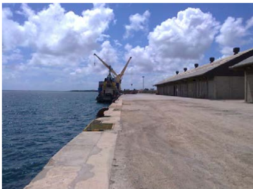
Photo 3.12: 383 m Long Straight Berth
