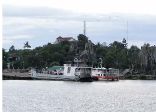
Photo 3.40: RoRo Jetty at Mwanza North Port
