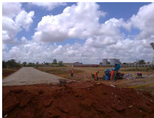
Photo 3.15: Future Container Yard under Construction
