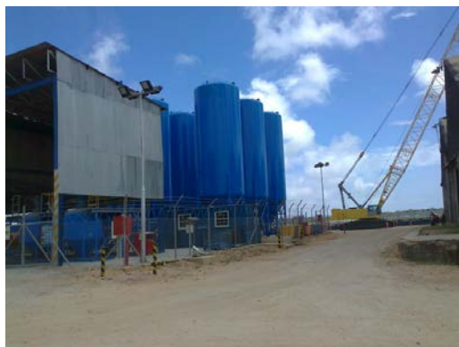
Photo 3.14: A Concessionaire of Oil and Gas Exploration Uses Part of the Berth
