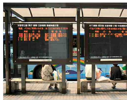
Figure 4-15 Example: Image of Bus Location Information Provided at Bus Stop
