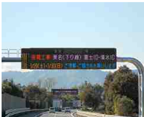
Figure 4-5 Example: Image of Variable Message Signboard
