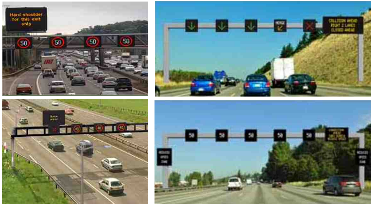
Figure 4-21 Example: Image of Lane Control by Showing Variable Speed Limit According to Time and Traffic Conditions in UK and USA
