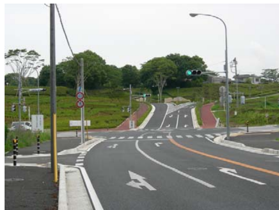
Figure 221 Intersection (2) in Japan
