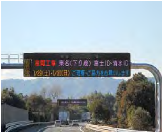
Figure 103 Variable Message Signboard
