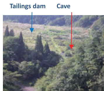
Tailings dam (H=85.5m)
