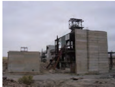
There are no safety fences for facilities
