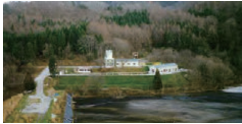
Tailings dam and Mine water treatment facility (Aomori Pref.)
