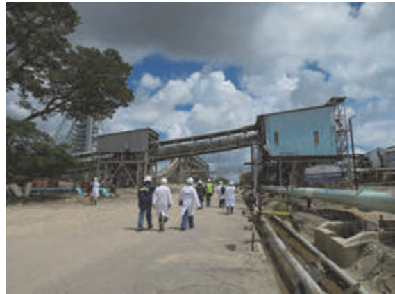
Photo 4.42 View of the Facilities (conveyor, mill and concentrator) in Konkola Mine
