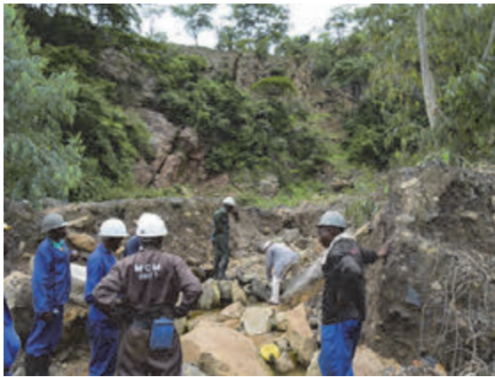
Photo 4.5 Outflow of Drainage Water from Former Mine Mouth and Collapse of the Upper Portion of the Mouth
