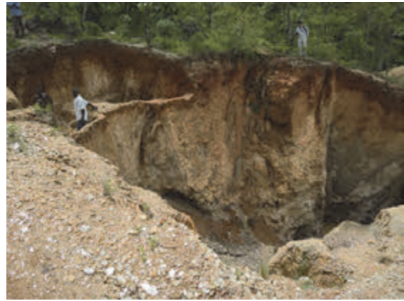
Photo 4.30 Condition of Digging Site (the shape shows trench-like)
