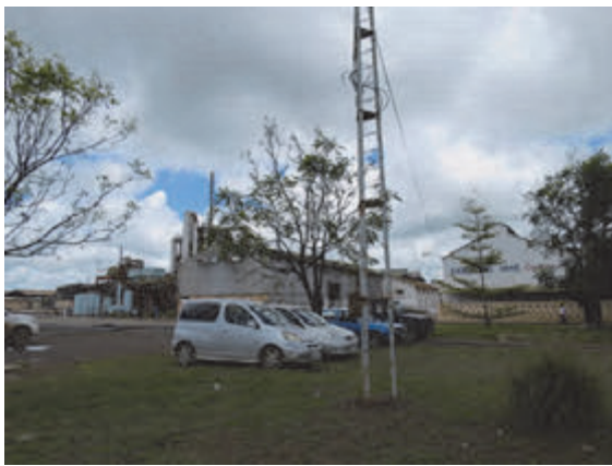
Photo 4.49 Entrance of Former Mine Facilities (Sable Zinc Ltd has been using the facilities.)
