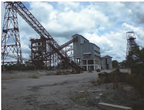
Photo 3.26 Primary crushing plant
