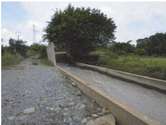
Photo 4.35 Spillway from Tailing Dam (directly flow in to diversion)
