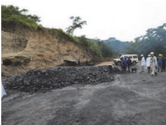
Photo 4.9 Condition of Mine Mouth
