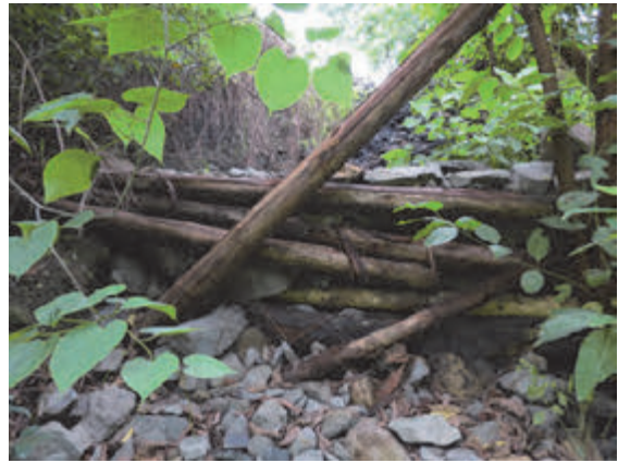
Photo 4.4 Drainage Filter by Stone Bond under the Crude Stock
