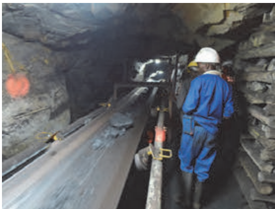
Photo 4.21 Condition of Walkway in the Drift of the Mchenga Coal Mine
