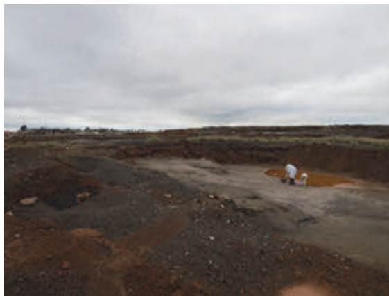
Photo 4.51 Former Tailing Dam (slag and waste were refilled at the time of closure.)
