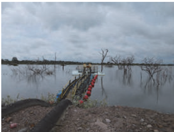
Photo 4.45 Water Pumping at Tailing Dam (the water used for industrial and domestic water near the tailing)
