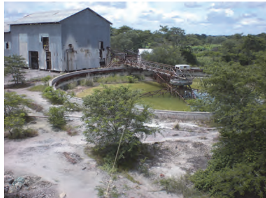
Photo 3.27 Concentrator and thickener
