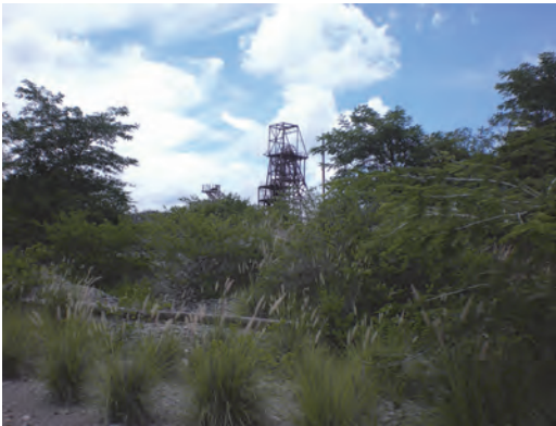
Photo 3.24 State of shaft and mining area
