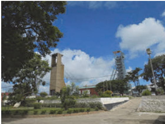
Photo 4.41 Shaft of Konkola Mine (right side is used for carrying crude ore from under ground)
