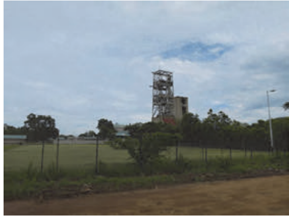
Photo 4.34 Shaft of Mopani Mine
