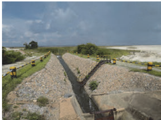
Photo 4.36 Spillway of Tailing Dam (directly flow in to diversion)
