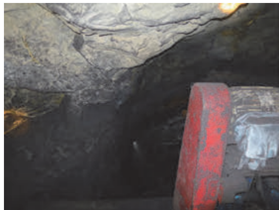
Photo 4.22 Condition of Roof in the Drift of Mchenga Coal Mine
