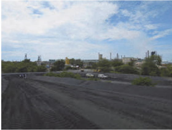
Photo 4.33 View of Facilities (shaft and smelter) of Mopani Copper Mine
