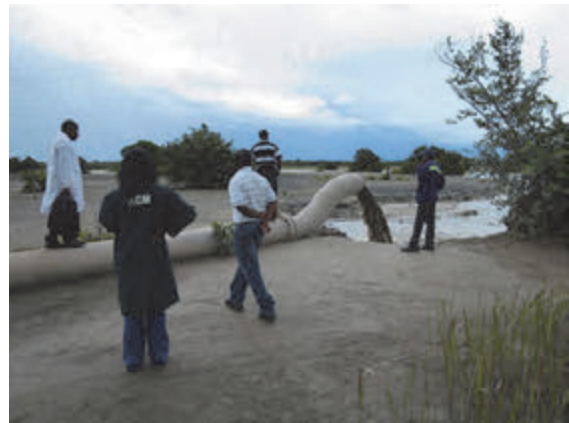
Photo 4.44 Discharge to Tailing Dam (tailings are conveyed by slurry pipe from the concentrator)
