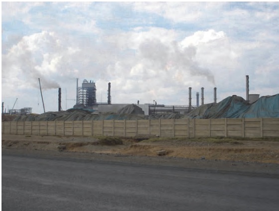
Photo 3.9 Smelter of Mufulira Mine in Copperbelt in Northwest of Kitwe City
