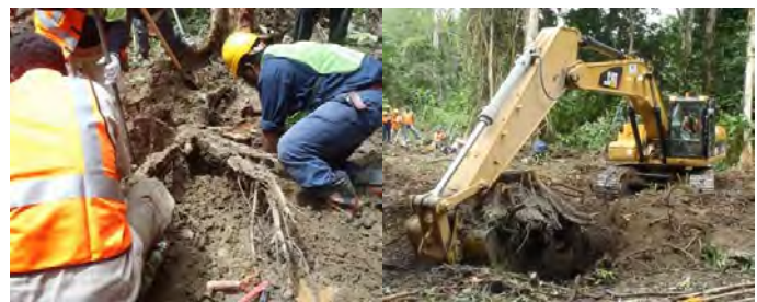
Digging roots by hand
