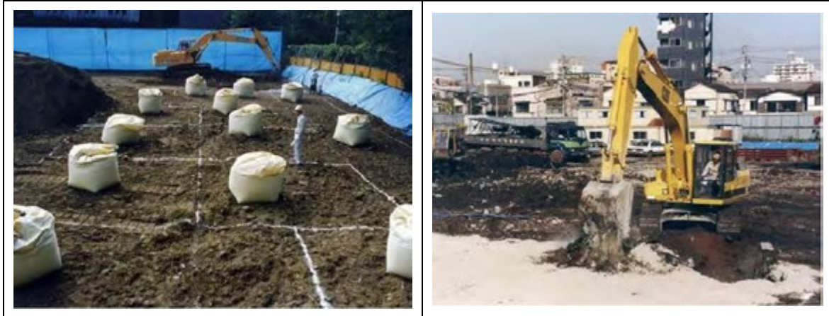
Figure 5.13 Construction Method of Cement Solidification Ash by Backhoe
