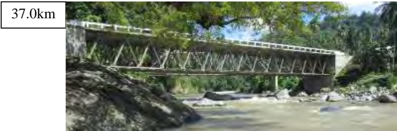
37.0km Uguiaban Bridge (Flood Deposit is not almost observed)
