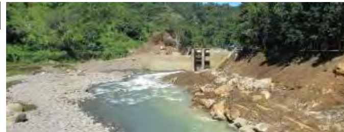
CEPALCO Dam (No Debris flow Deposits)
