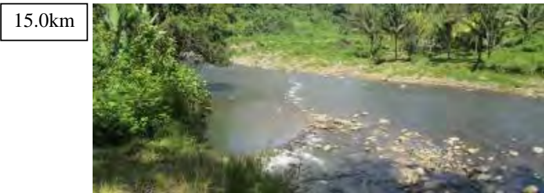
Mand Steel Bridge (No Debris Flow Deposit)
