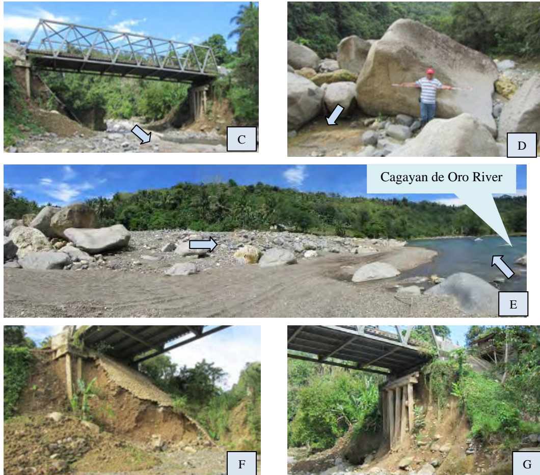
Photo 3.2.20 Condition of the Debris Flow (Bitanog River) (2/2)
