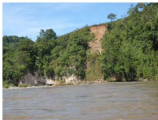
Surface Failure (CDO River 2012)
