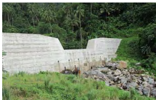
Check Dam in Camigin Island
