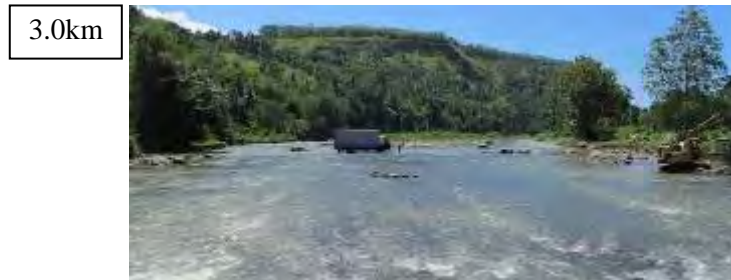
Tumalaong Causeway (Riverbed Covered with Gravel)
