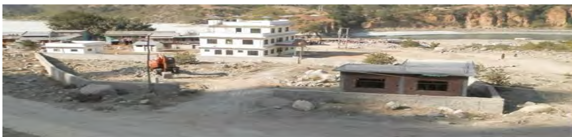
Collection Center under construction at Kurkhot (December 2013)
