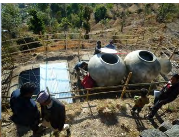
Multiple Water Utilization System (MWUS) supplying both for farming and domestic use
