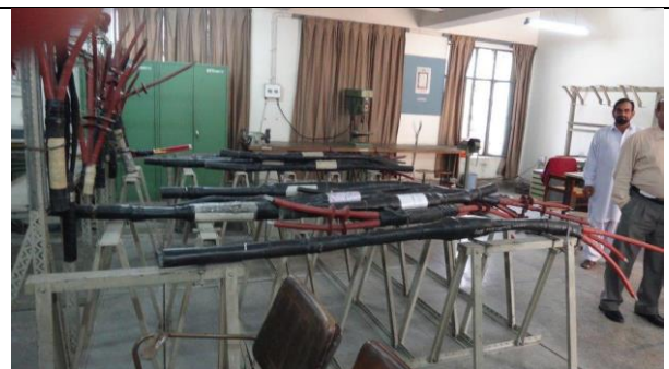
Cable Joint Training
