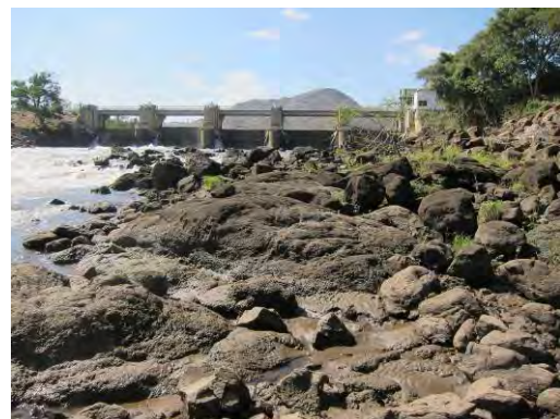
Photo-4: New Intake Site
