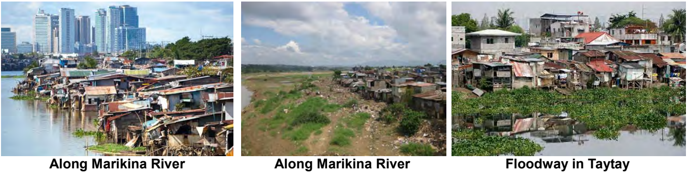
Source: MMDA, Preparatory Study for Sector Loan on Disaster Risk Management (JICA, 2010), Your One Voice,
