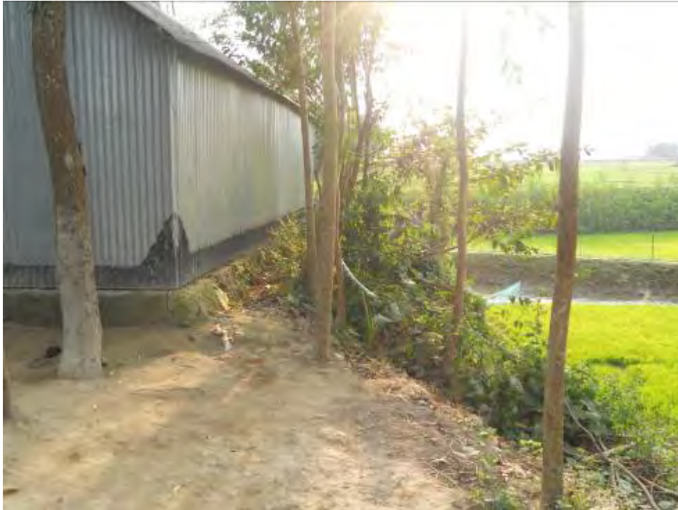
Photo: Affected housing structure of Md. Abul Kalam Village:Protimabanki;Mouza: Protimabanki; Pourashava:Sakhipur; District:Tangail
