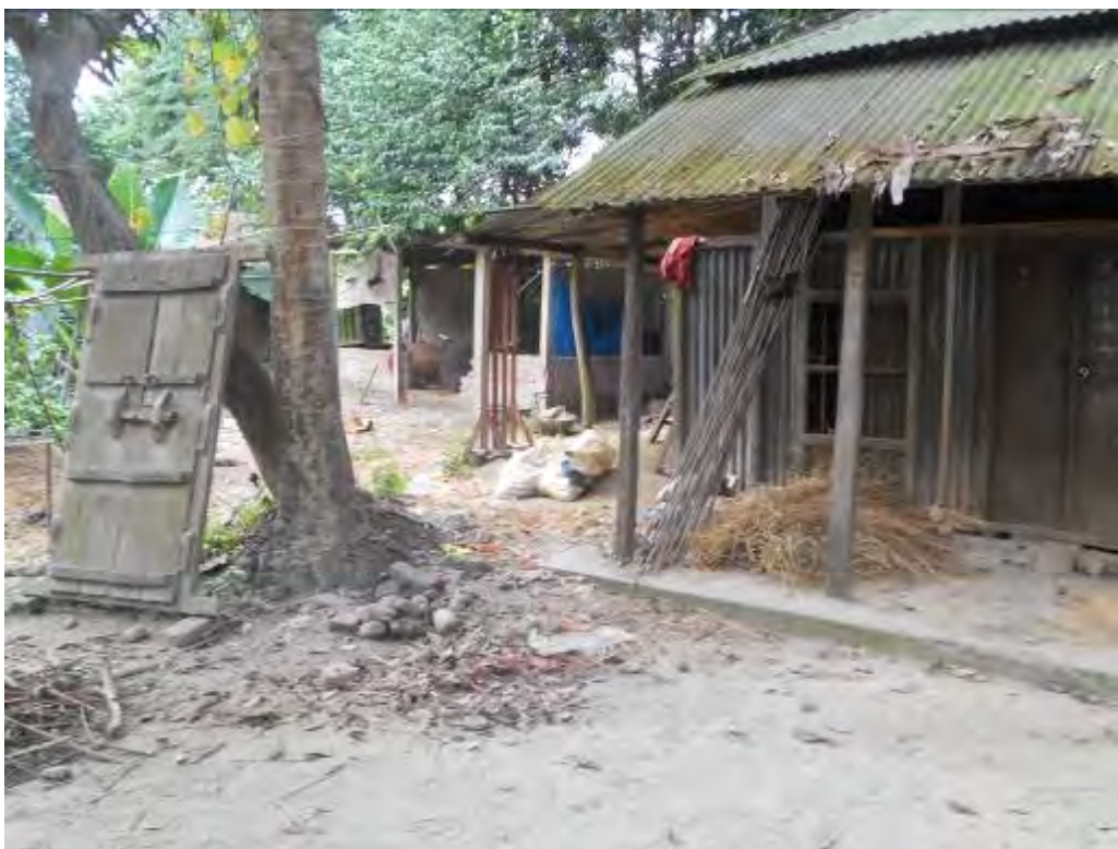
Photo: Affected household Structure of Humayun Kabir, Village : Mohish jora; Mouza: Mohishjora, Union: Bukdahara: Upazila: Kalihati; District: Tangail
